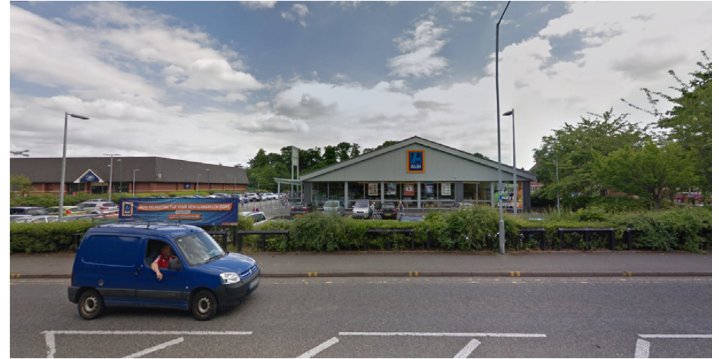
4.0 Fig. 2 View of the existing shopfront from the Retail Park Access Road.
