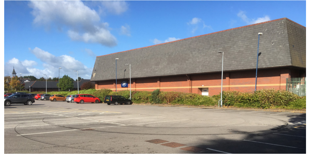
4.0 Fig. 6 View of adjacent retail unit's relationship with the existing store.
