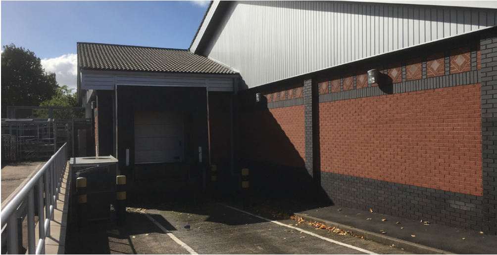
4.0 Fig. 5 View of the existing dock leveller service point.
