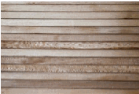
Example of Cedar Cladding (Timber Cladding)
