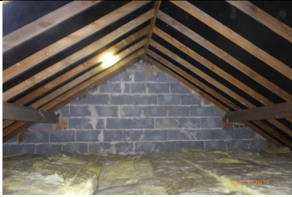
Photograph 9: Loft void of building 7.
