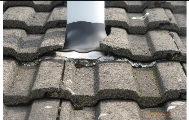
Photograph 12: Bat roost feature identified within building 7.
