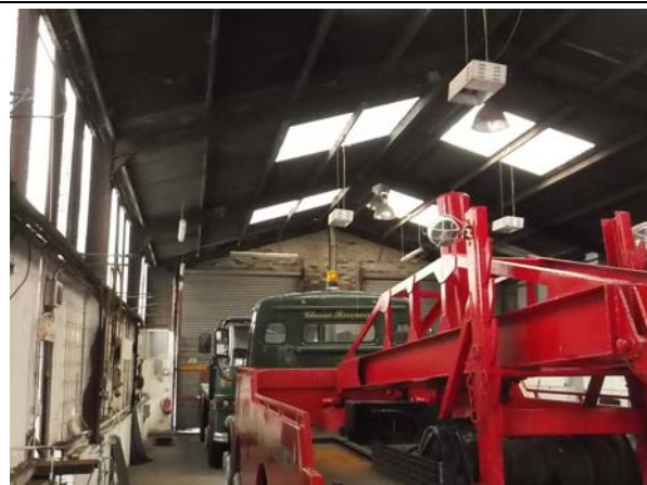
Photograph 6 – Interior of Building 5
