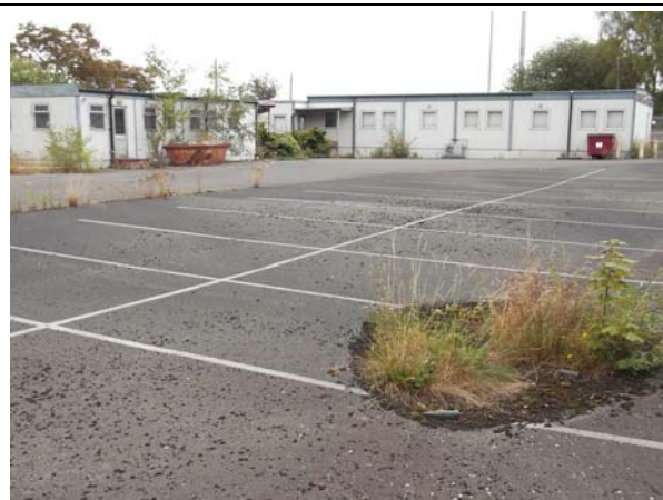
Photograph 8 – Hard-standing yard areas
