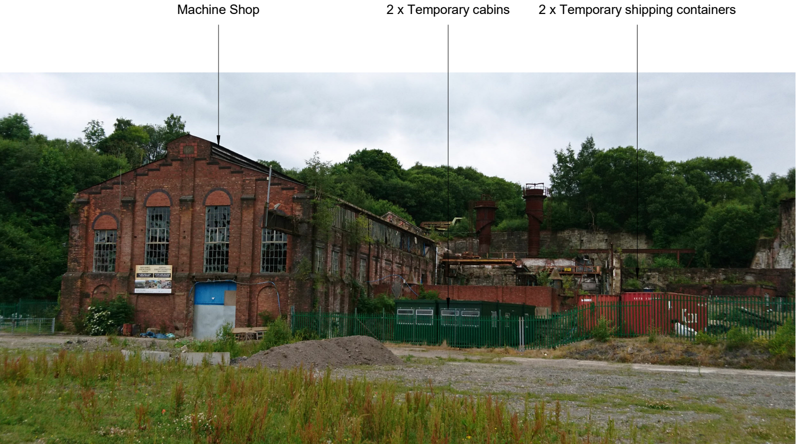
View of temporary structures from front of site
