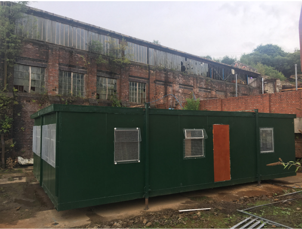
2 x Temporary cabins on site - dimensions 9.8m x 3.1m each
