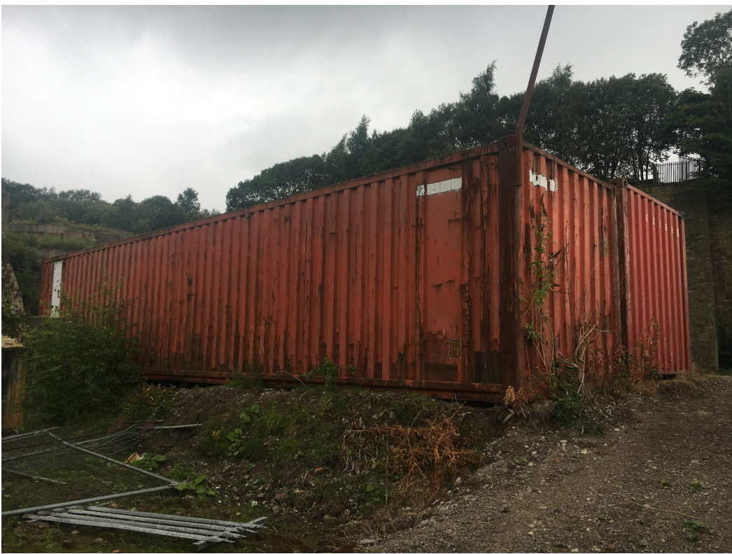
2 x Temporary shipping containers on site - dimensions 12.4m x 3.4m each
