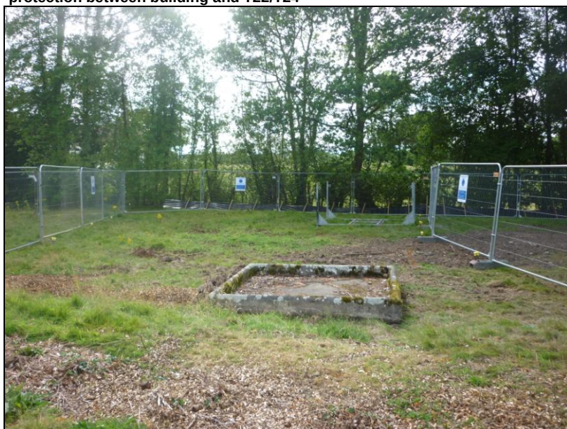
Photo 10 - Tree protective fencing erected around T24/G10
