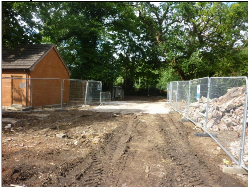
Photo 13 - Tree protective fencing erected around T30-32 & W1 from access of internal road
