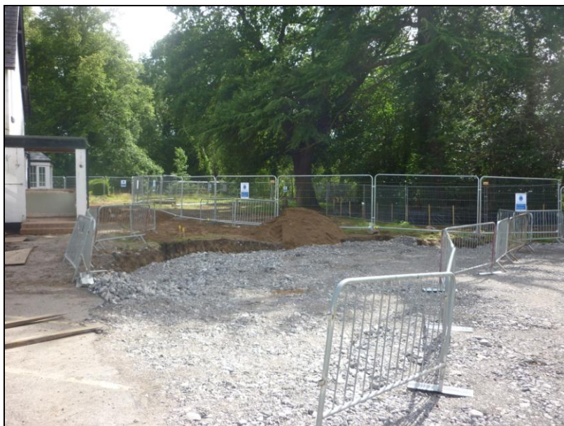
Photo 8 - Tree protective fencing erected around T21-T24
