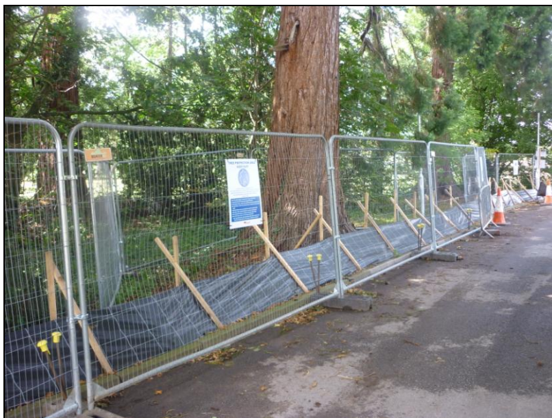
Photo 1 - Tree protective fencing erected along western edge of main access road in accordance with Tree Protection Plan (TPP)
