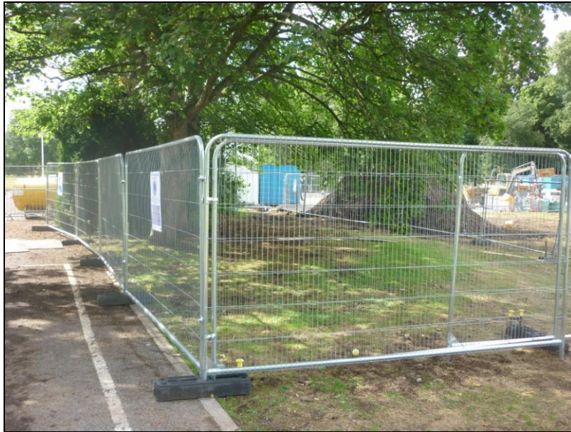
Photo 18 - Tree protective fencing erected around TG14
