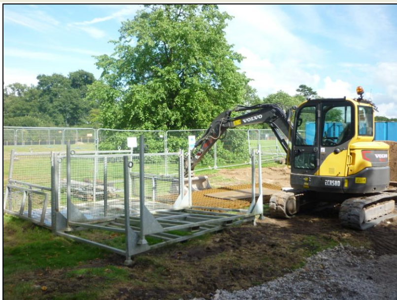
Photo 6 - Tree protective fencing erected around T11
