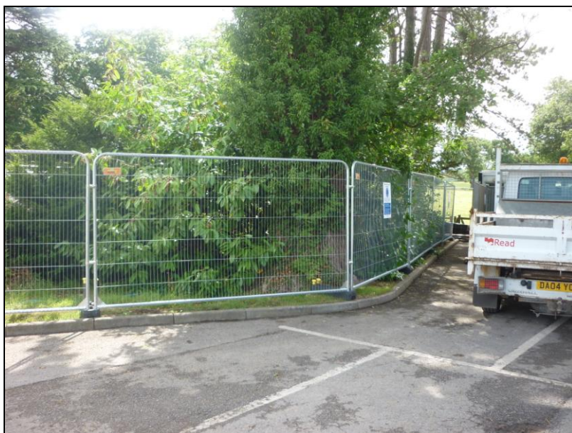
Photo 7 - Tree protective fencing erected around T18 as per TPP
