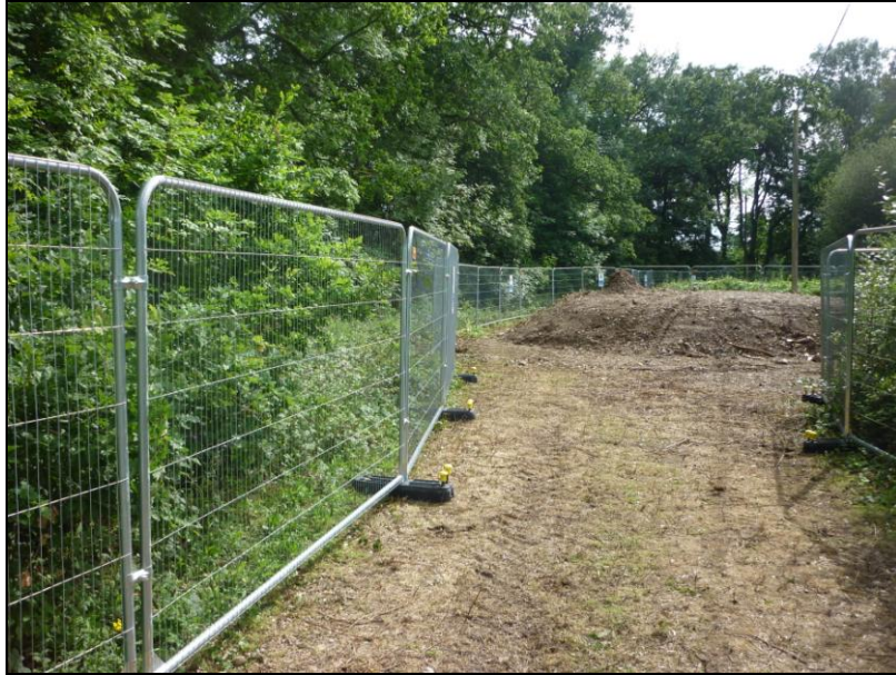
Photo 12 - Tree protective fencing erected around proposed spoil mound area in SE corner of site. Mound located outside RPA of trees and a 1.5/2m easement is to be retained between the mound and fence along eastern boundary
