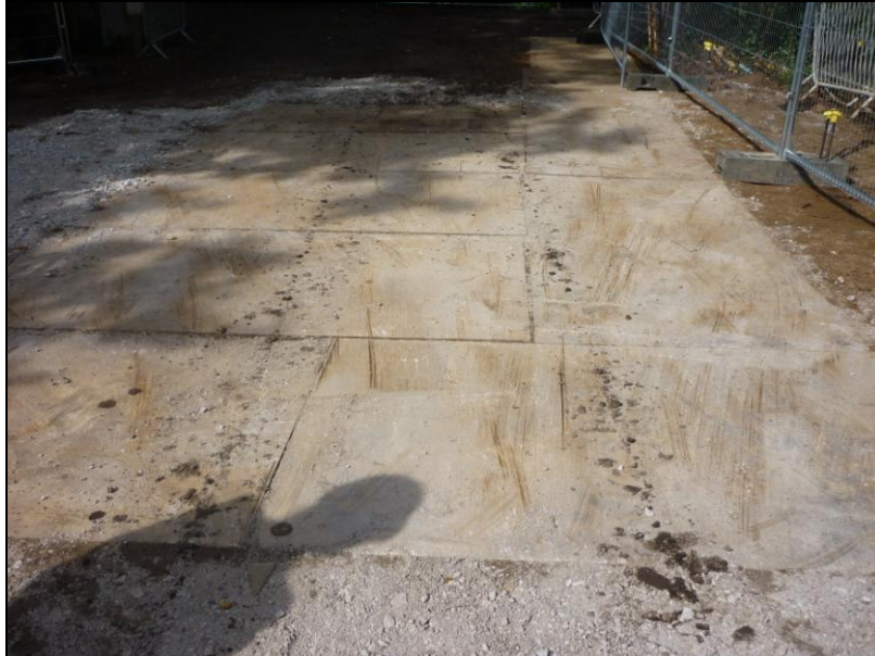
Photo 15 - Steel plate ground protection laid upon compressible layer of sand. Type 1 roadstone laid around edge of boards - section towards T32 to be removed
