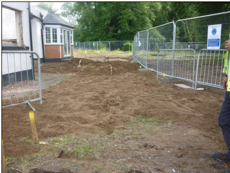
Photo 9 - Sand laid in preparation for installation of bog mat ground protection between building and T22/T24
