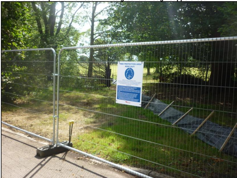
Photo 5 - Tree protective fencing erected in front of G8
