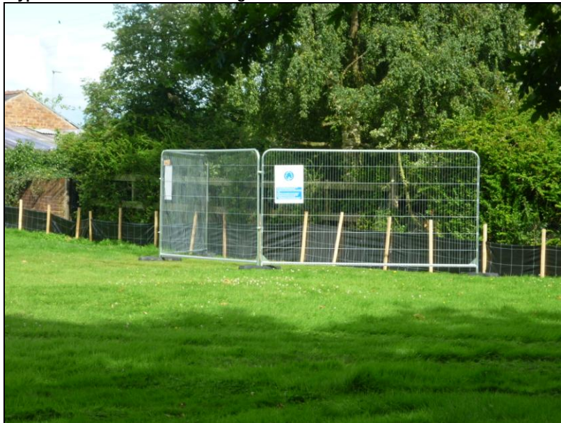
Photo 16 - Tree protective fencing erected around T1 to prevent soil mounding within RPA
