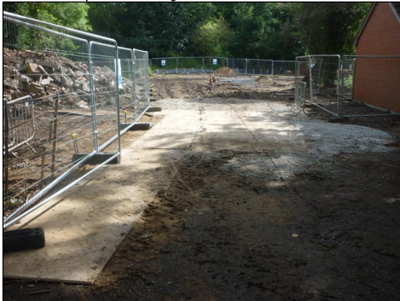
Photo 14 - Ground protection (steel plates) installed between T30 & 32 as per AMS
