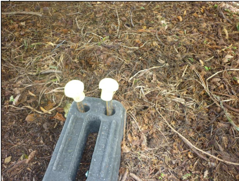
Photo 3 - Steel pins driven 500mm into ground through support feet
