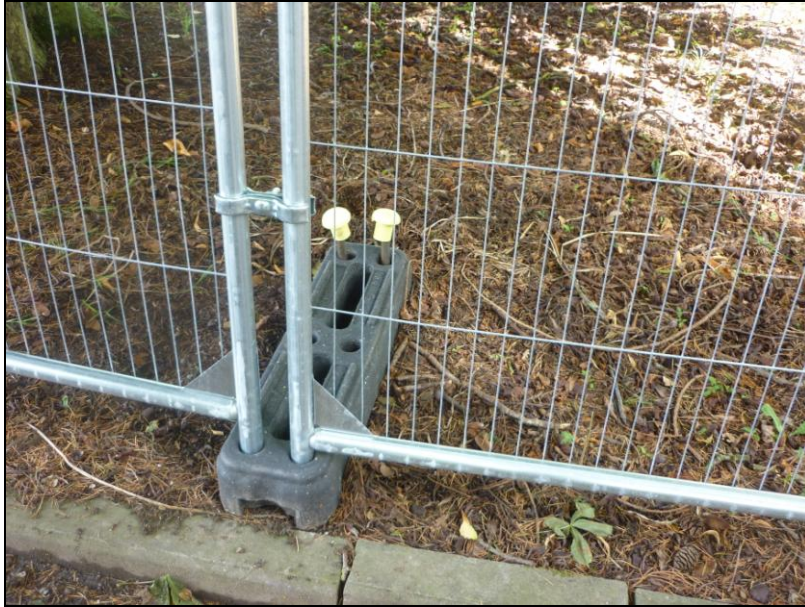
Photo 3 - Heras fence panels supported in plastic footing and fixed firmly in place by steel pins driven into the ground. Each panel is connected by anti-taper bolts and cannot be moved
