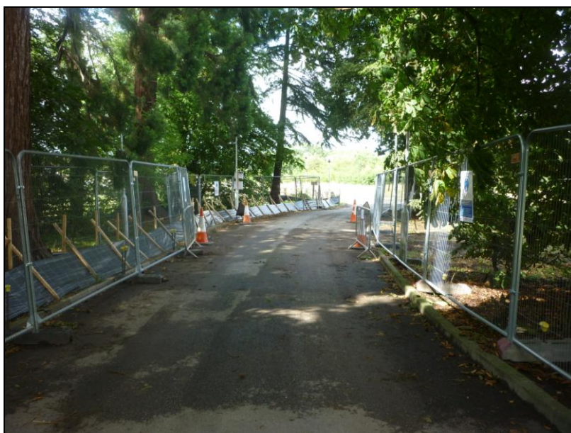
Photo 2 - Tree protective fencing either side of access road
