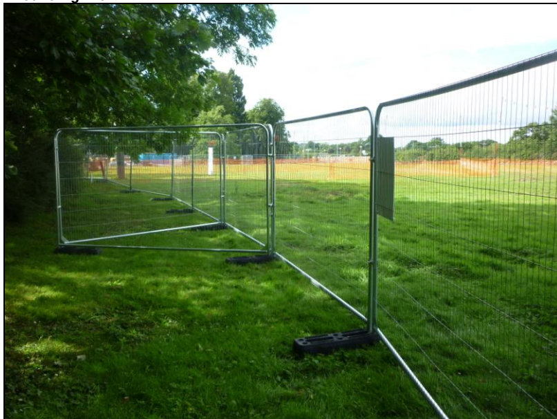
Photo 17 - Tree protective fencing erected around G13 & G14 - protection during excavation of lake
