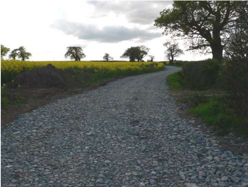
Photograph 5: Upgraded access track alongside hedge and ditch
