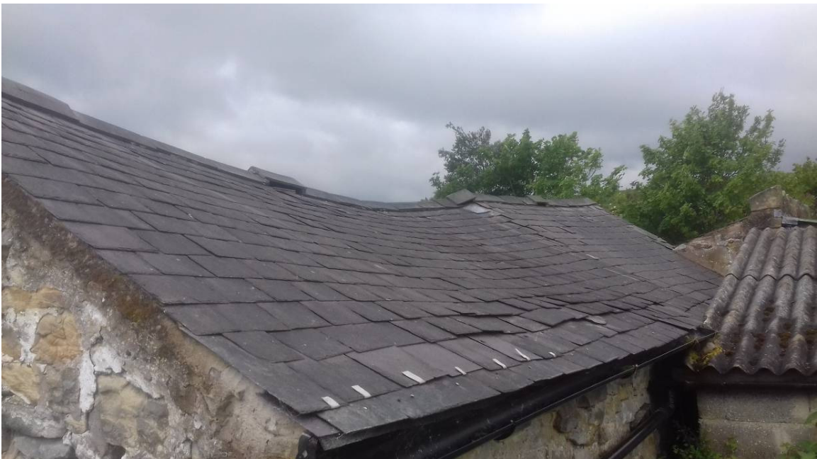
Southern roof elevation of O1
