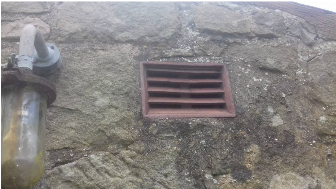
Ventilation to western elevation of O1
