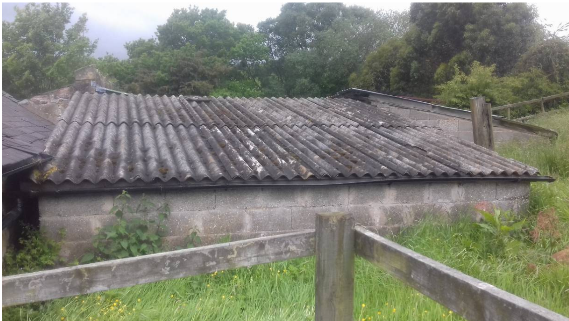
Rear elevation of O2
