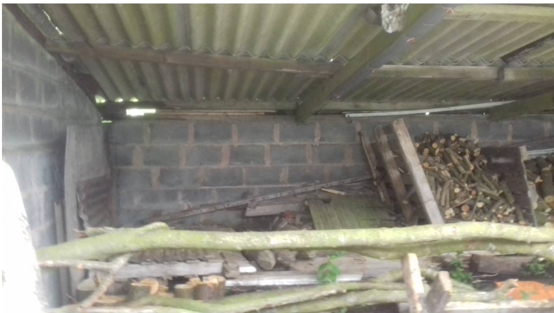
Interior of O3 with part asbestos part metal corrugated roof – no potential
