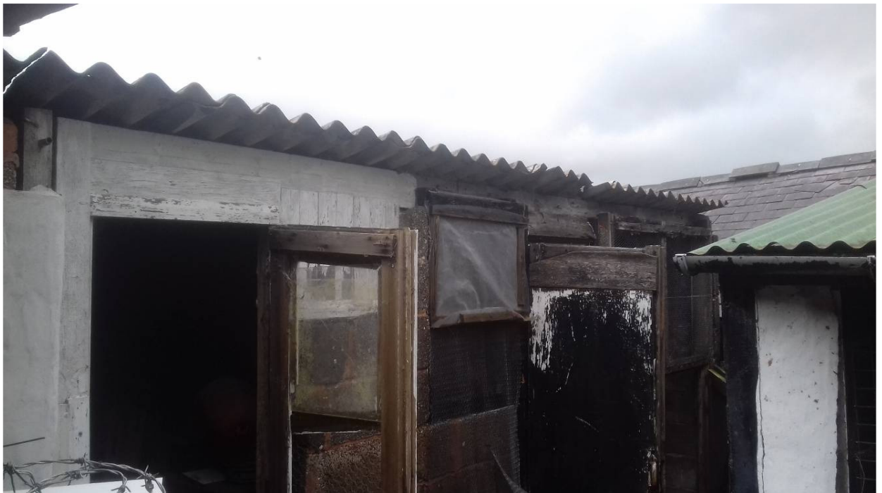
Front elevation of Outbuilding 2 (O2)
