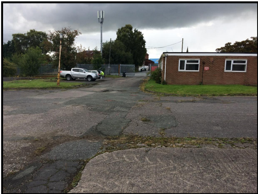
8. Looking south at the building in the central south of the site.
