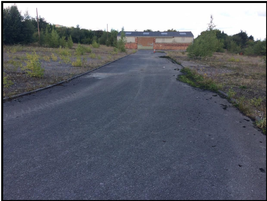
10. Looking north at the east of the site.
