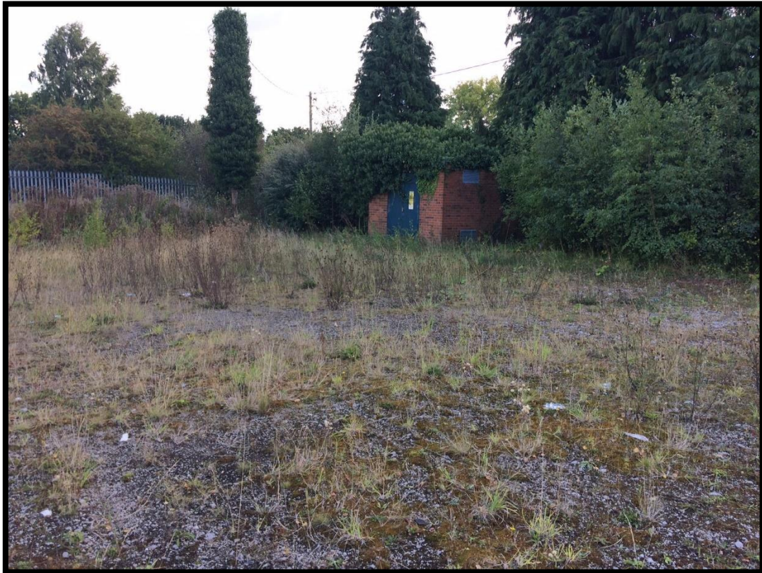
11. Electricity sub-station in the south east of the site.
