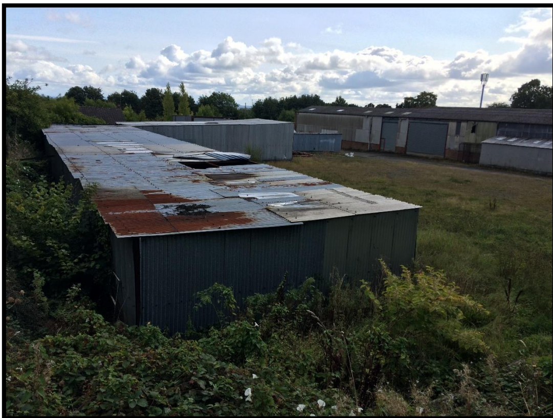
1. Looking east over the north of the site.
