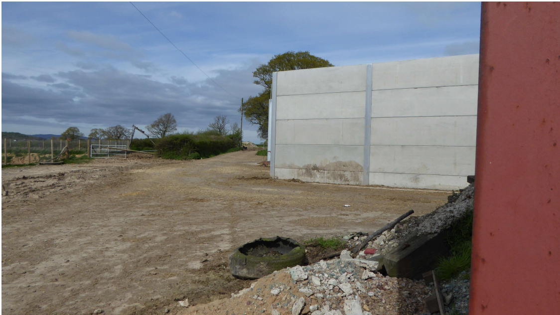
4. View from South looking north – rest of clamp is screened by existing building.
