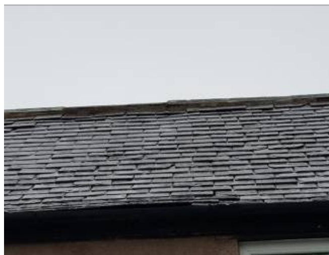
Roof of B1
