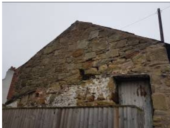
Exterior wall of B3
