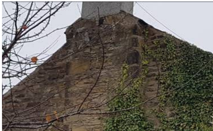
Exterior stone wall of B1
