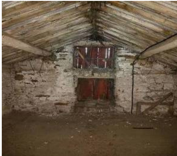
Interior of B2
