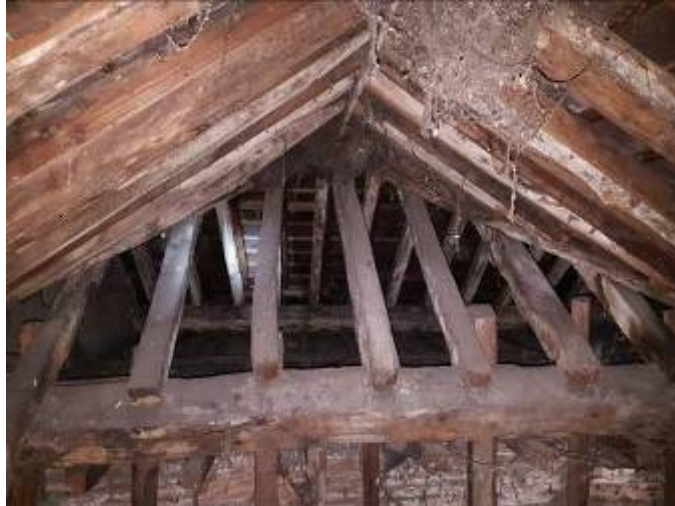
Section joining two loft spaces (B1)
