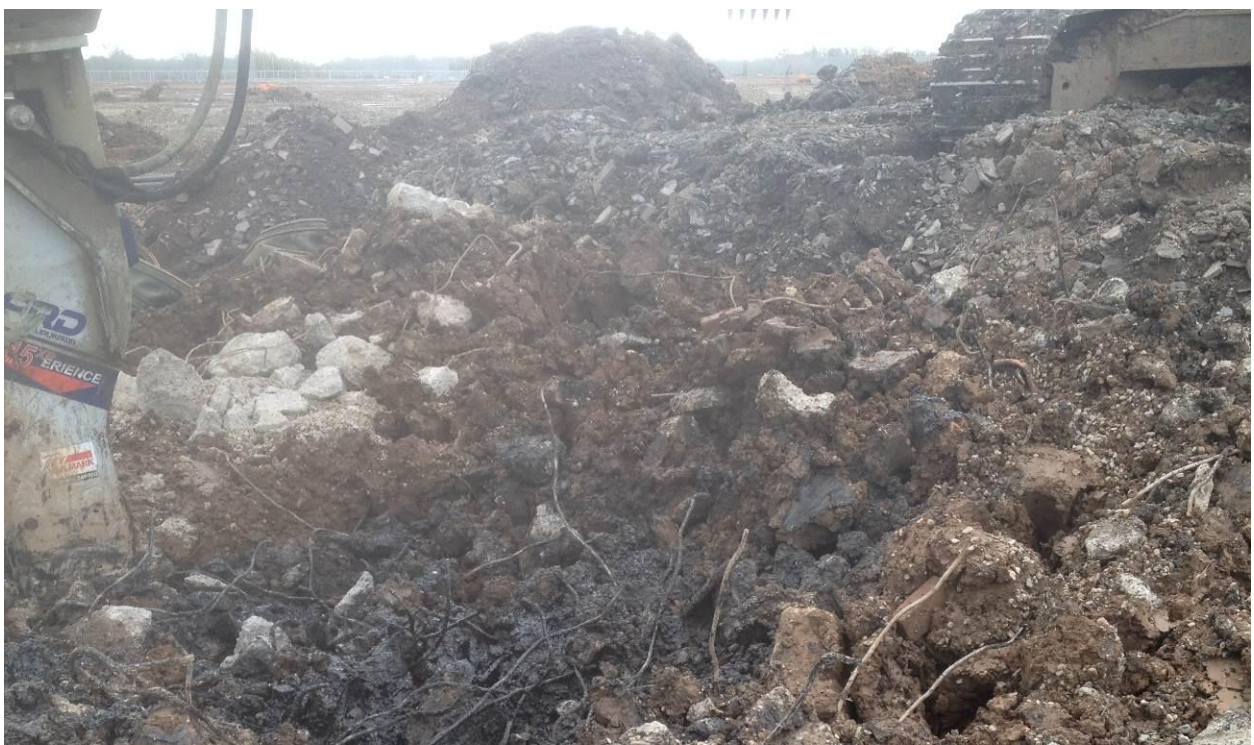
Figure 8: Location of ATP2 showing black 'resin' material.
