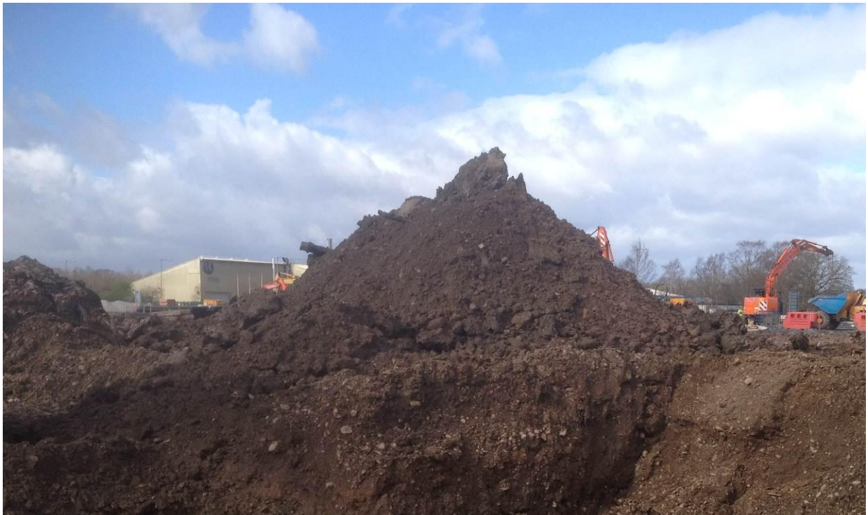
Figure 7: Excavated material stockpile in which sample SP1-SP3 were taken.
