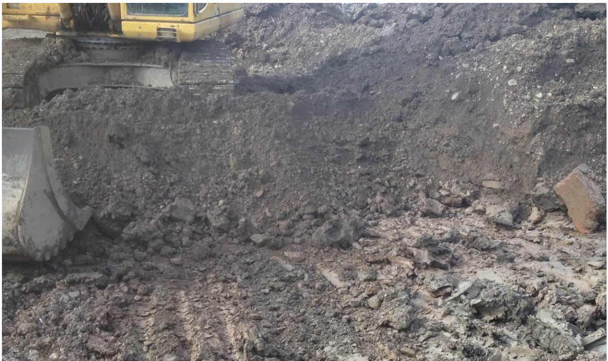
Figure 2: Southwestern edge of 'soft spot' excavation where S4 was taken.
