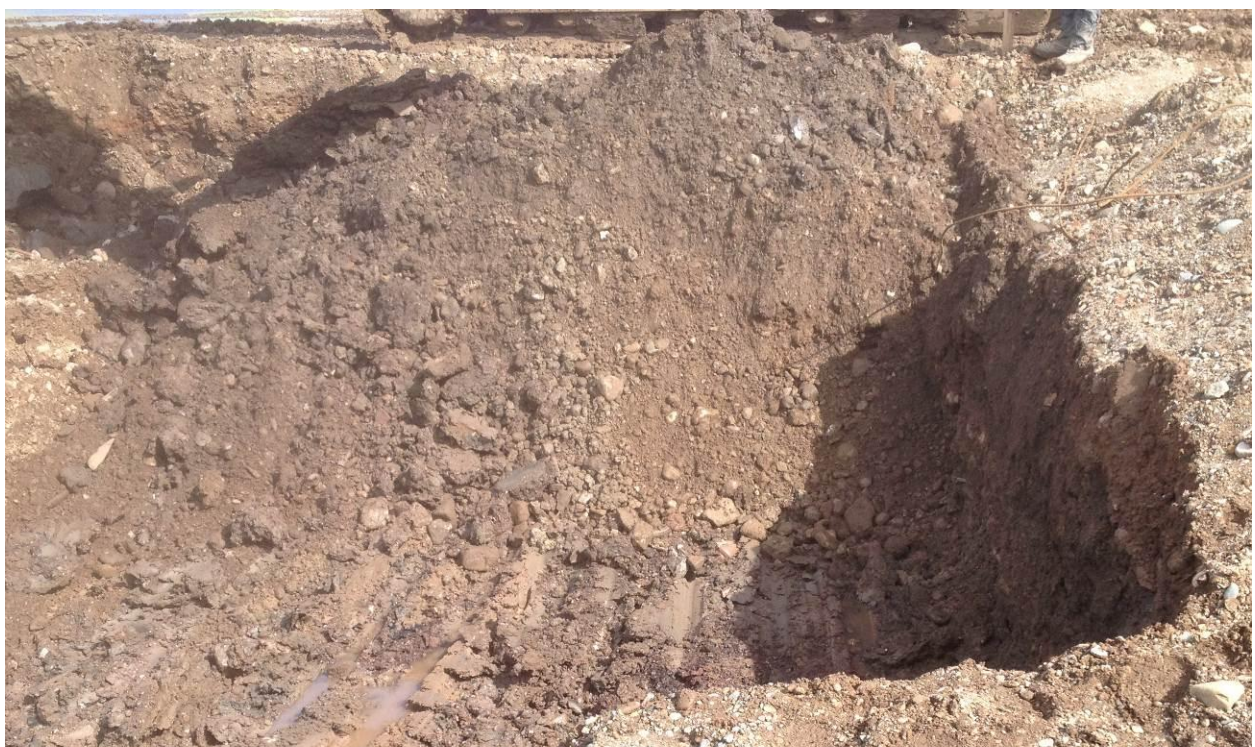
Figure 4: Southeastern corner of 'soft spot' excavation where S1 was taken.
