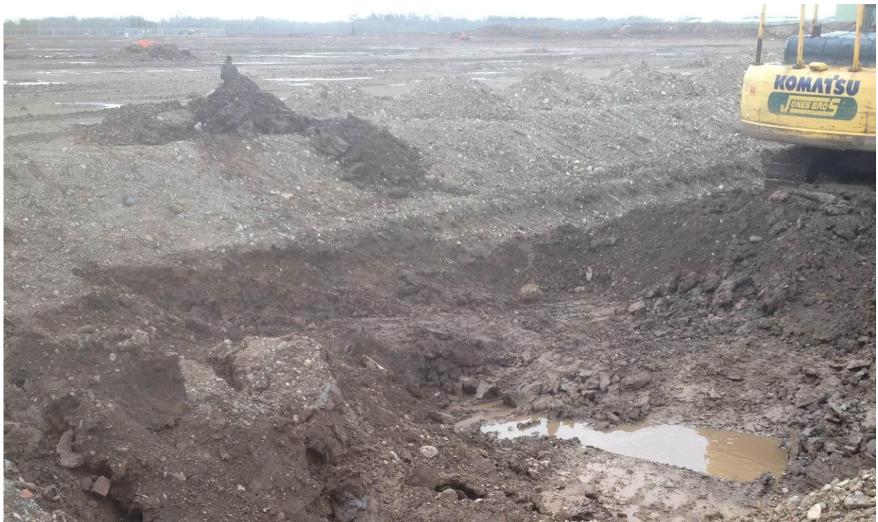
Figure 3: Southeastern edge of 'soft spot' excavation where S6 was taken.
