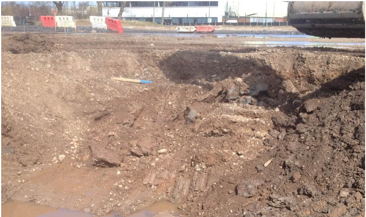
Figure 5: Northeastern edge of 'soft spot' excavation where S2 was taken.
