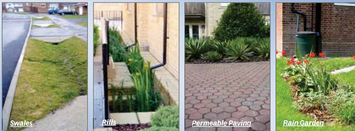
Figure 6: SuDS Photographs (SusDrain, 2012)
