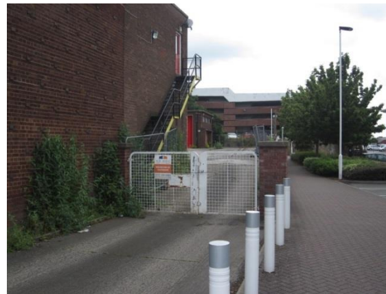
Fig 4: View of access to rear of site.
