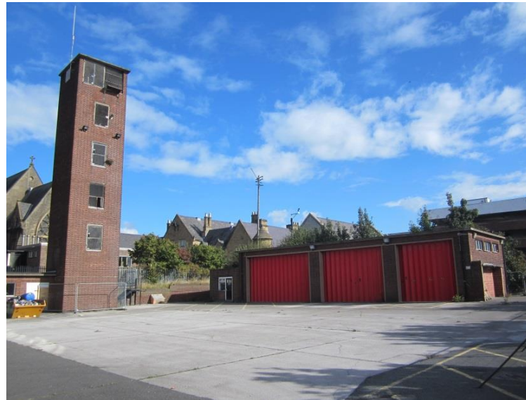
Fig 6: Fire station yard with tower to north boundary and mechanic's shop to east boundary with Cathedral, Museum and Multi storey car park beyond.
