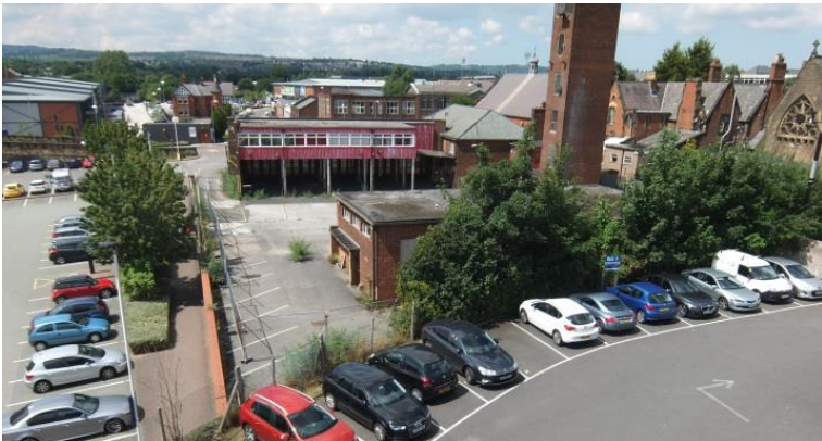
Fig 1: View of site from existing multi-storey car park.
