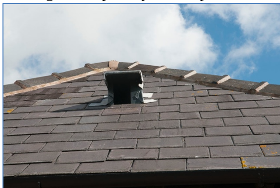
Photograph 3: A Habitat entrance had been placed on the western side of the roof.
