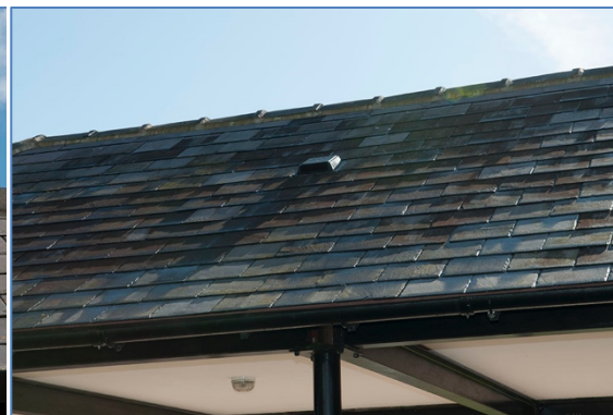
Photograph 4: There is also an entrance on the northern side of the roof.
