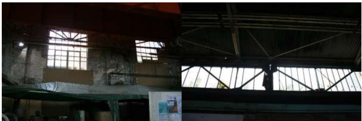
PICTURE 5. OLD CRANE PROVIDING ACCESS TO THE GABLE
