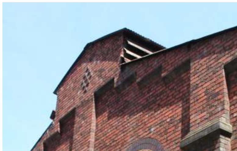
PICTURE 3. VENTS ON THE GABLE END
