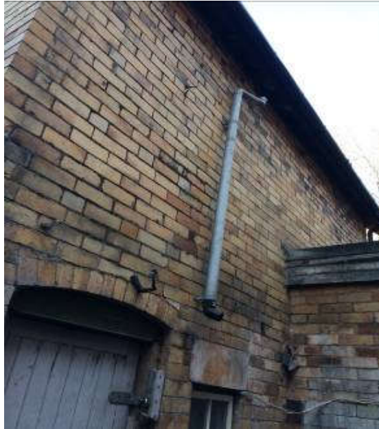
Side elevations where eaves are open.
