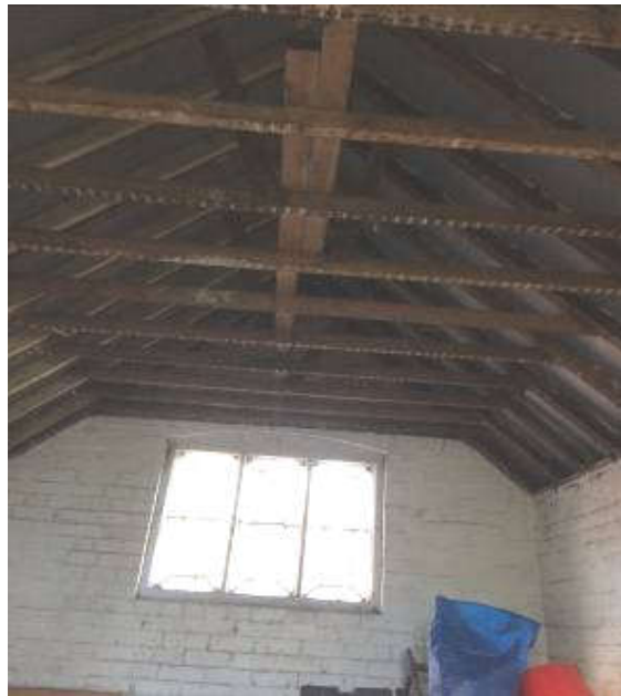
Interior with ceiling removed and breathable membrane evident.
