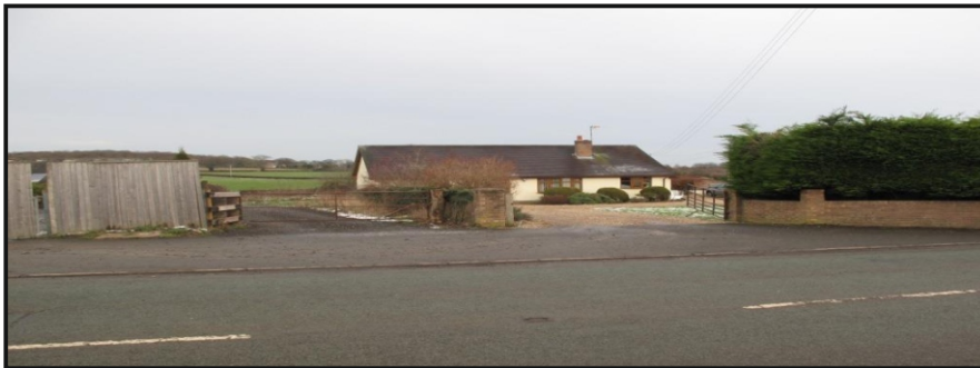
Existing entrance to Area A ▲
