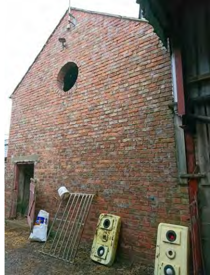
Photo 3 – Outbuilding Rear Elevation.
