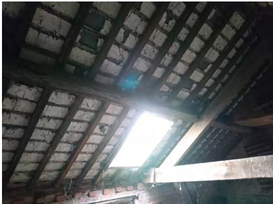
Photo 13 – Typical condition of roof construction
