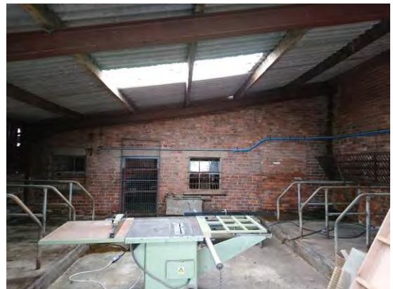
Photo 4 – Outbuilding Rear Elevation within covered area.
