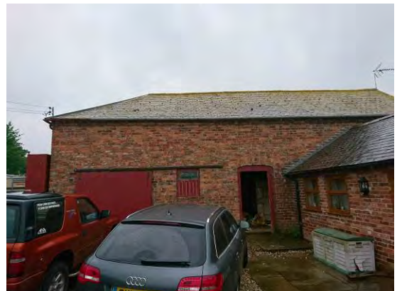
Photo 5 – Outbuilding Right Hand Side Elevation.
