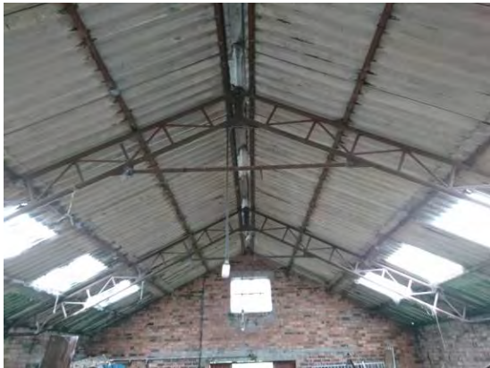
Photo 18 – Typical view of roof construction.
