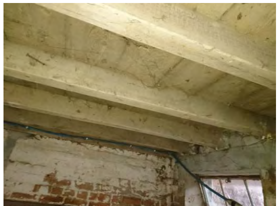
Photo 10 – Typical condition of first floor construction.
