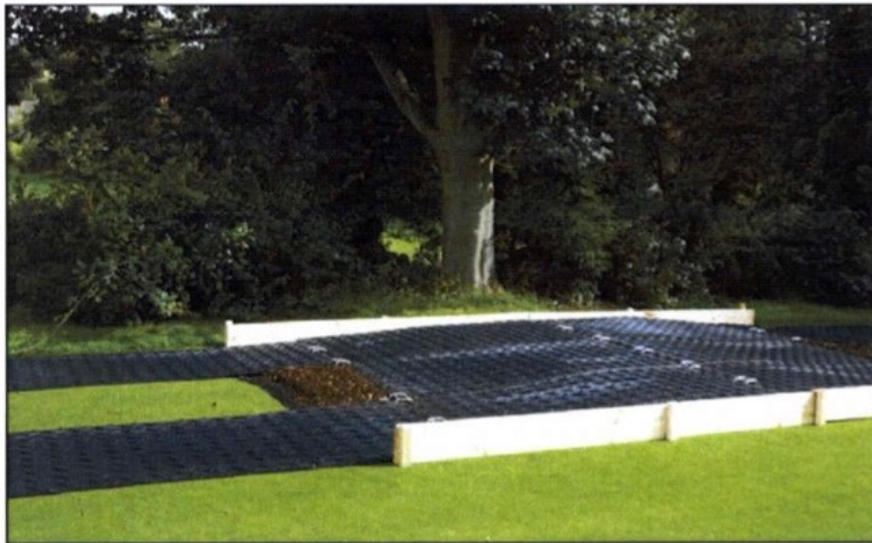
Green Tek Ground Guards showing geotextile membrane, 100 mm of woodchip with panels above to protect tree roots
