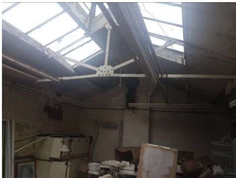
Interior of glass roofed section
