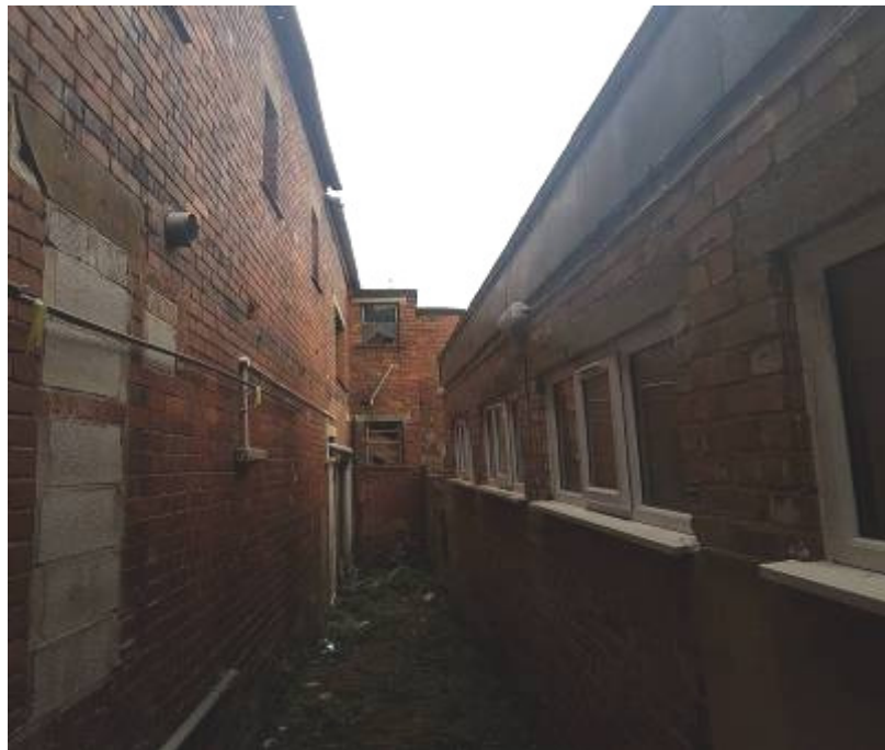
Side elevation of three storey section at the rear
