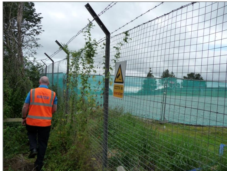
Figure 4. Perimeter security fencing
