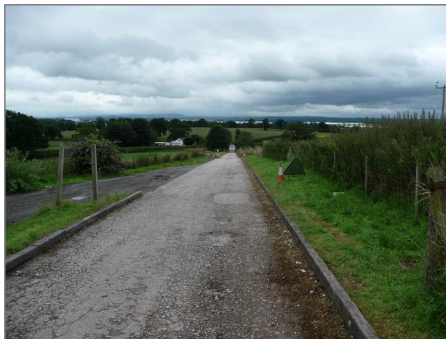
Figure 10. Access road to site
