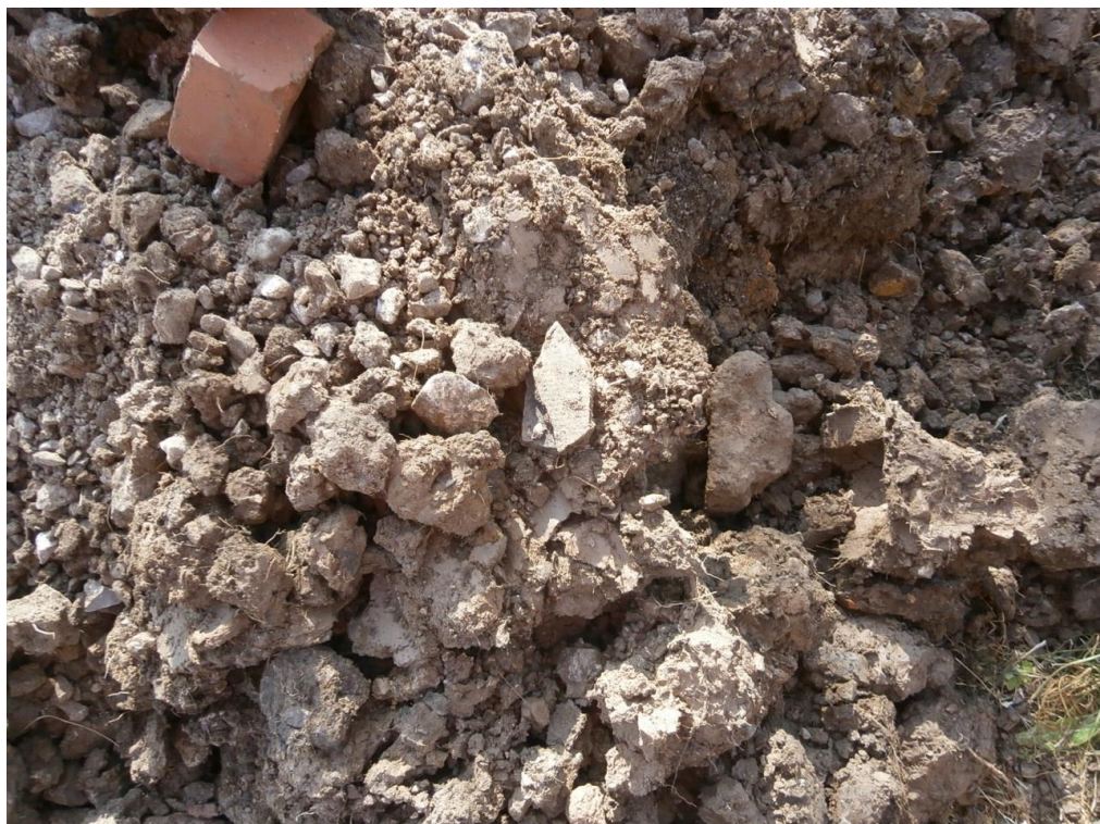
Figure 2: P1180021: Fragment of cement bonded asbestos prior to removal by litter-picking
