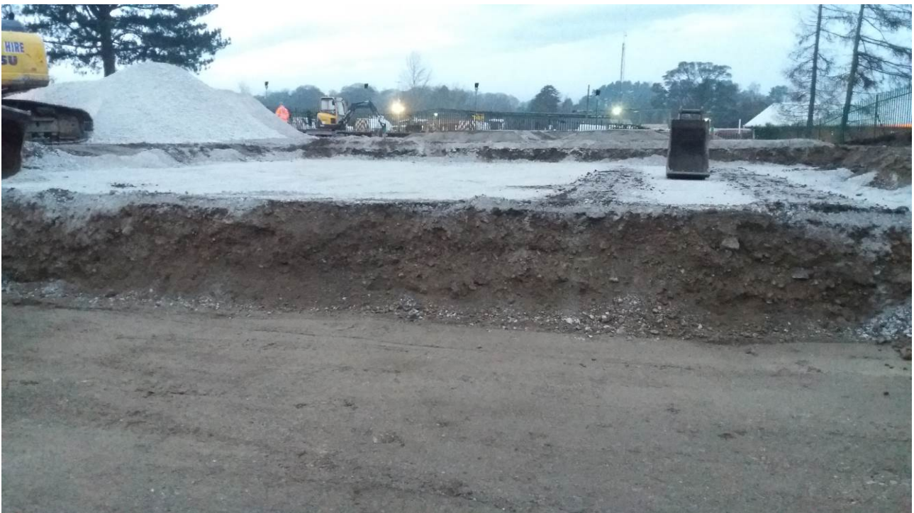
Photograph 1 Plot 7/8 showing the made ground comprising sand and gravel as proved by the site investigation
