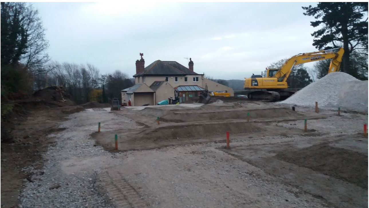
Photograph 6 showing plots 5 to 7
