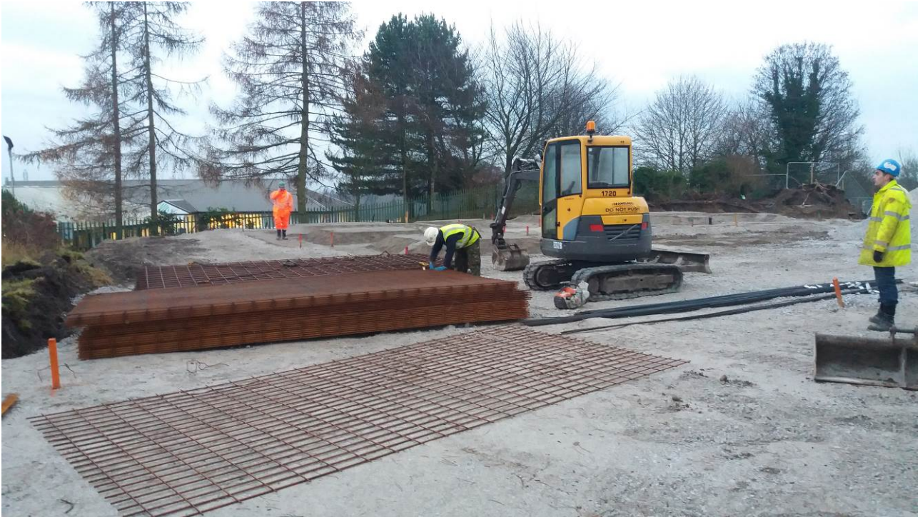
Photograph 2 Area A1 on left
