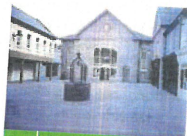
25 Listed Buildings at Bethel Square, Brecon
