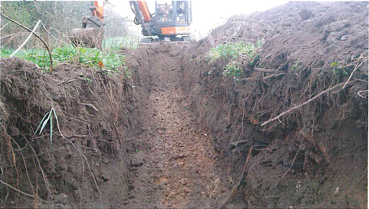
Photographs 8 Trench looking towards CH 22
