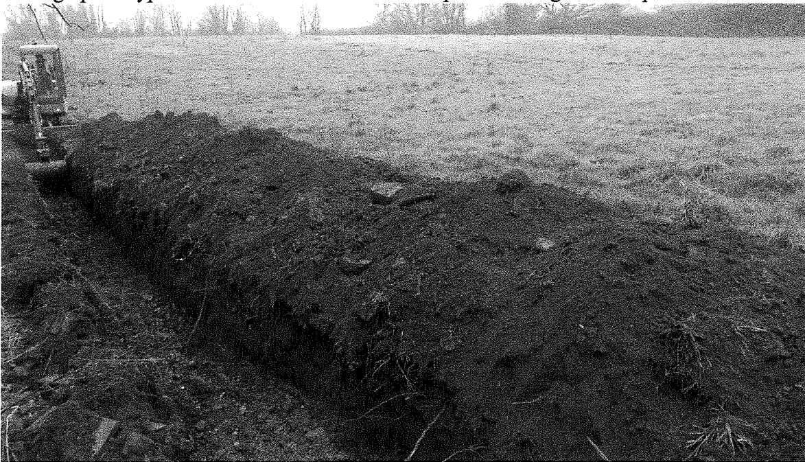
Photographs 6 showing spoil from excavation
