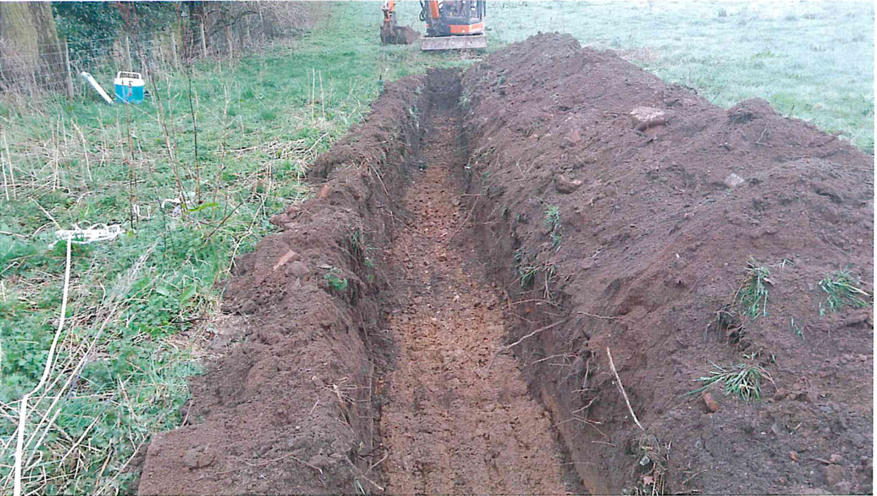
Photographs 4 Trench from CH 0 to CH 22
