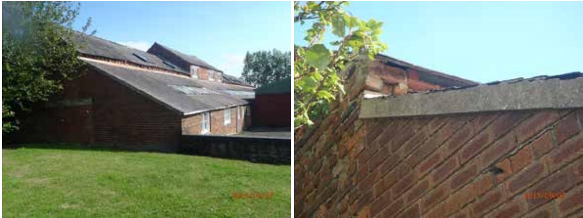
Plates 1a & 1b: View of Building 2 (TN1) with potential access points for bats
