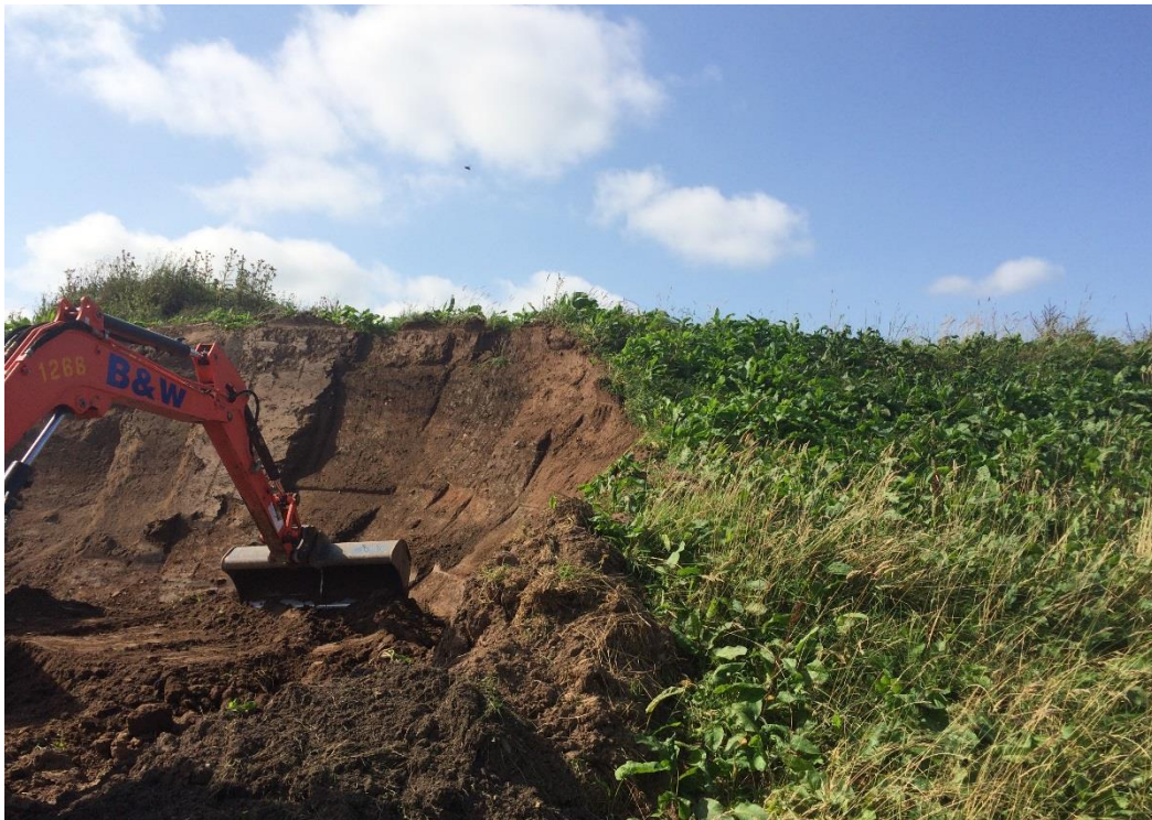
Plate 1: Looking along the southeast extent of the stockpile
