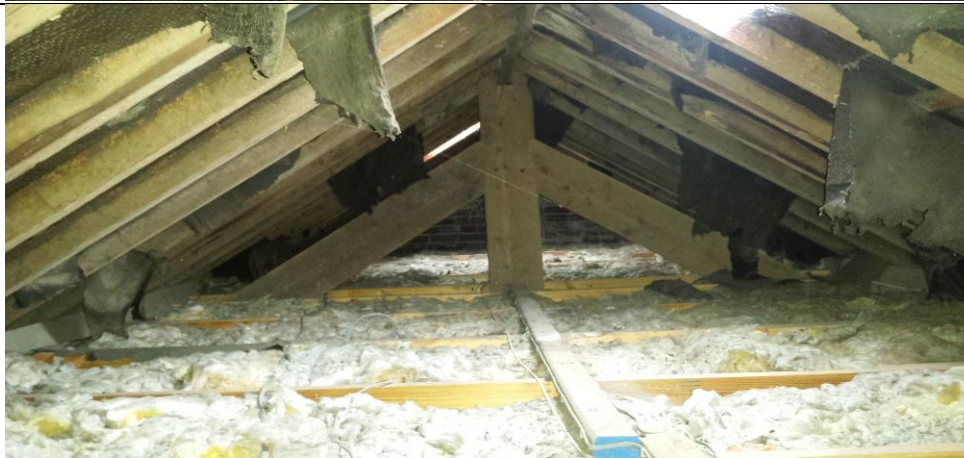
Photo 2: Interior of loft space in B1
