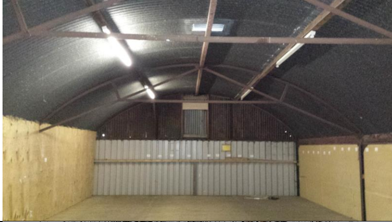
Photo 4: Interior of loft space B2
