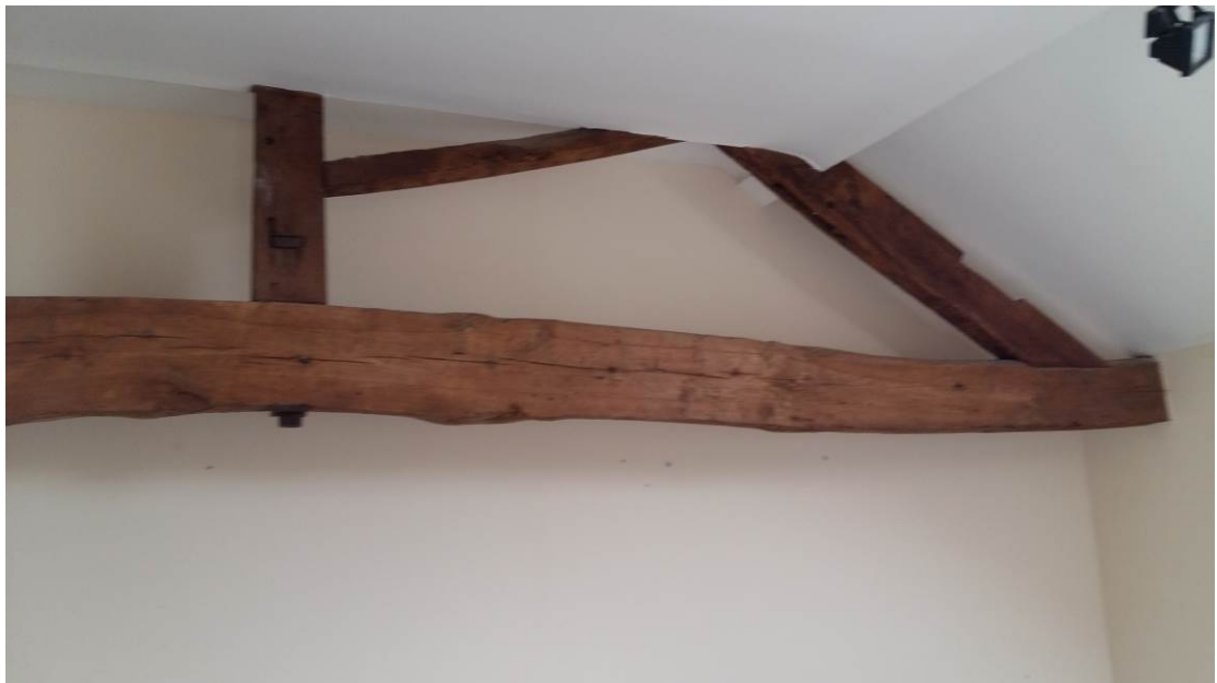
View showing roof trusses to be retained on first floor
