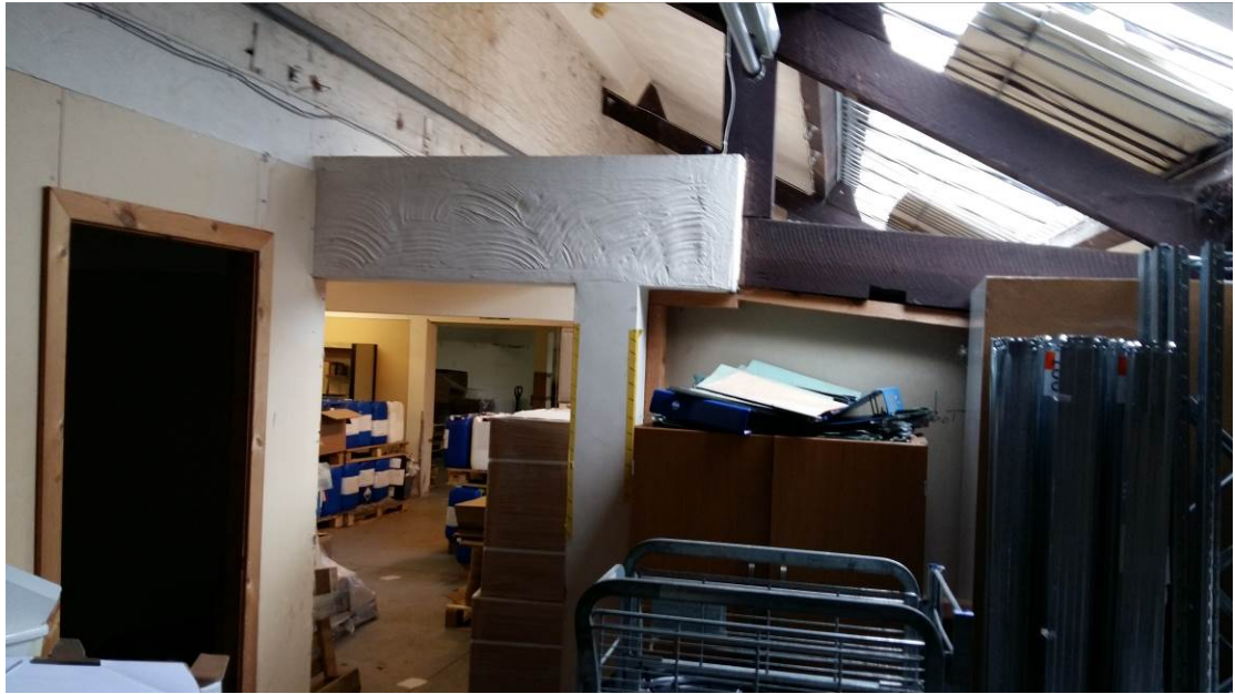
Views showing large structural elements
