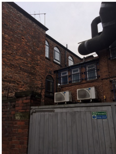
Photograph 8 - View from the cut-through : Rear elevation of Nos 14 & 15, High St
