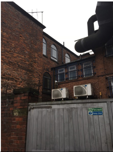
Photograph 4 - View from within the cut-through: Rear/side elevation of 20 High Street.
