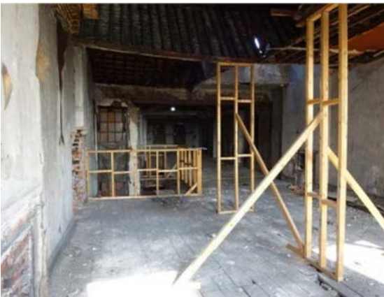
Photograph 13 – inside 20 High Street
