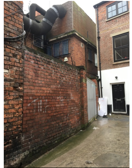
Photograph 3 - View from within the cut-through: Rear elevation of 20 High St
