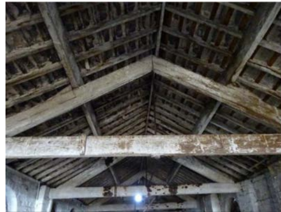
Photograph 12 – inside 20 High Street
