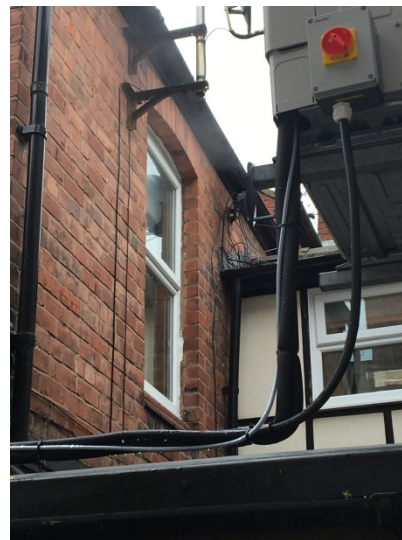
Photograph 16: First floor of the Wynnstay Apartments
