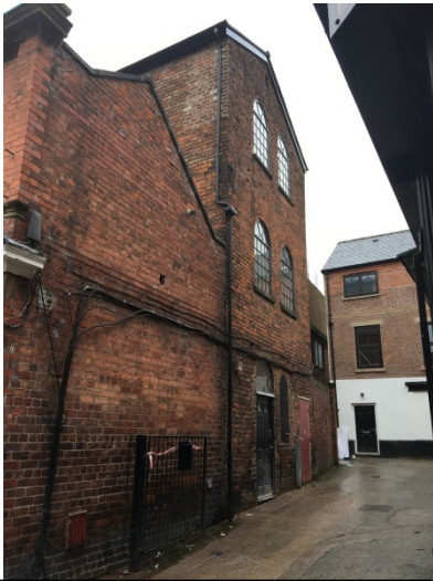
Photograph 1 - View looking west from Chester St: Rear elevation of 20 High Street.
