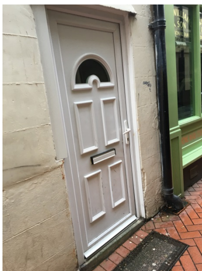
Photograph 17: UPVC door on Bank Street.
