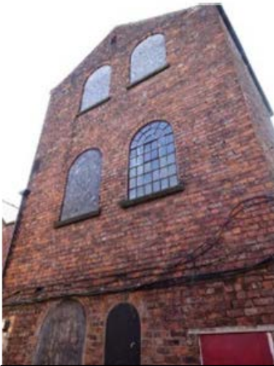
Photograph 9 – rear elevation (north) with boarded up windows
