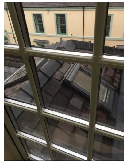
Photograph 6 - View from inside the building onto Chester St
