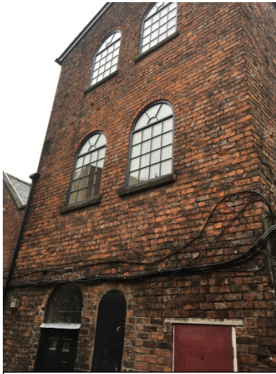
Photograph 2 - View from within the cut-through: Rear elevation of 20 High St
