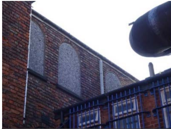
Photograph 10 – west elevation with boarded up windows
