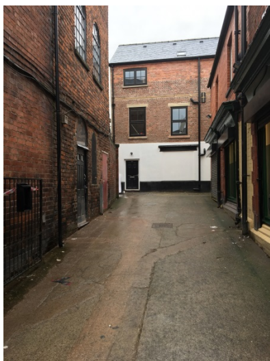
Photograph 14: 2a High Street
