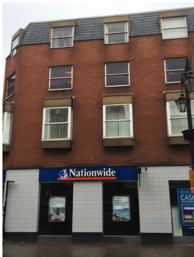
Photograph 20: UPVC windows at 1-2 High Street
