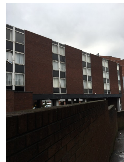
Photograph 19: UPVC windows at the rear of the Wynnstay Arms Hotel
