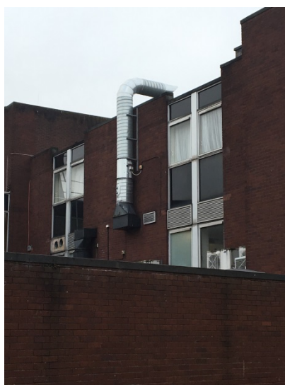
Photograph 18: UPVC windows at the rear of the Wynnstay Arms Hotel
