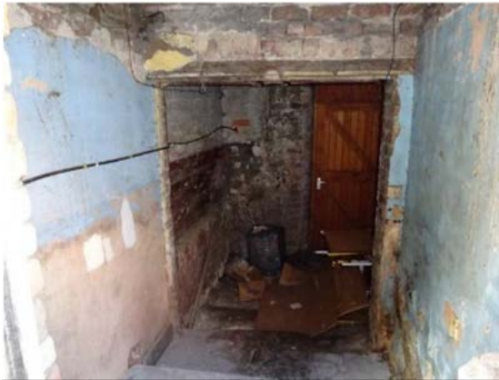
Photograph 11 – inside 20 High Street
