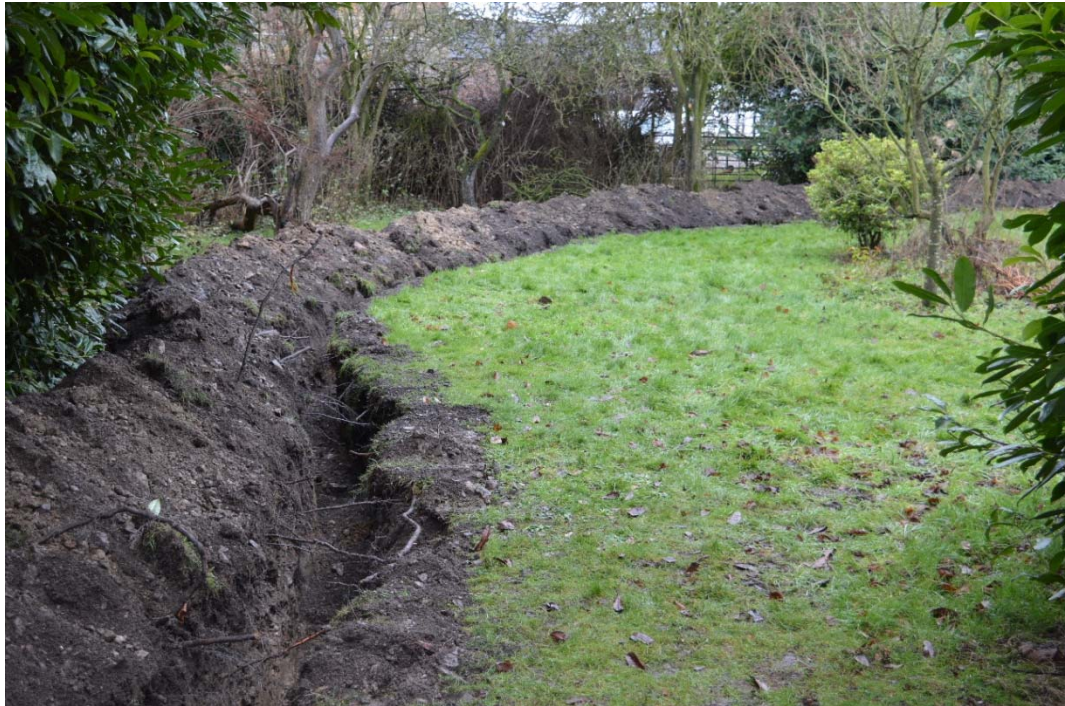
Fig. 5. The pipe trench to the south-east of the moat. Photo CPAT 4286-0001
