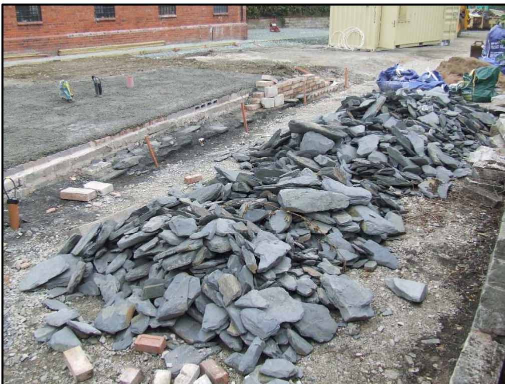
Photograph 10 Quarry slate to be used as stone facing to the station platform
