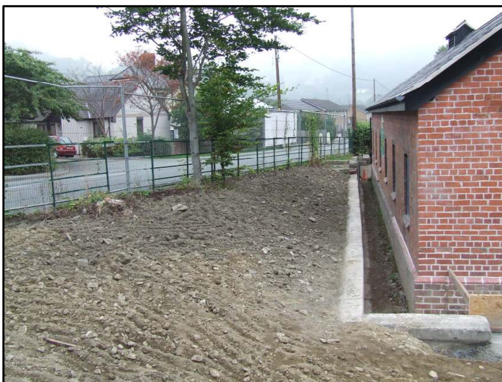
Photograph 6 Retaining wall and soils cleared of vegetation to the north of the old tram shed
