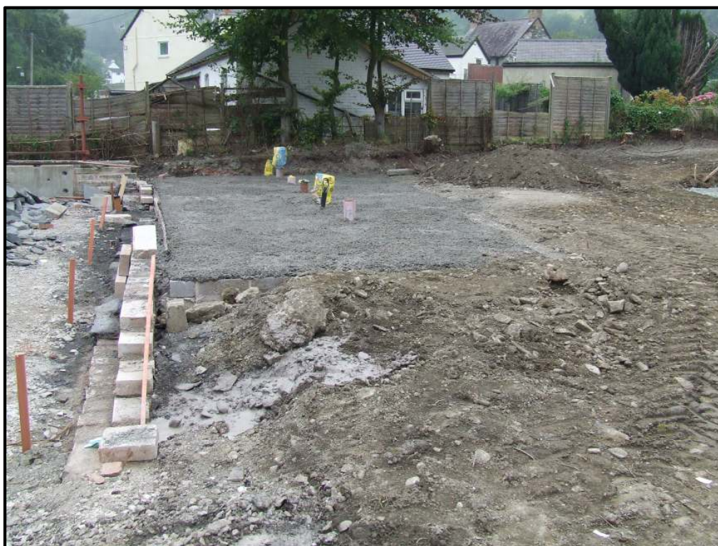
Photograph 7 Construction of the station platform in progress showing outline of wall forming the repository for soils elevated in PAHs, with concrete cap
