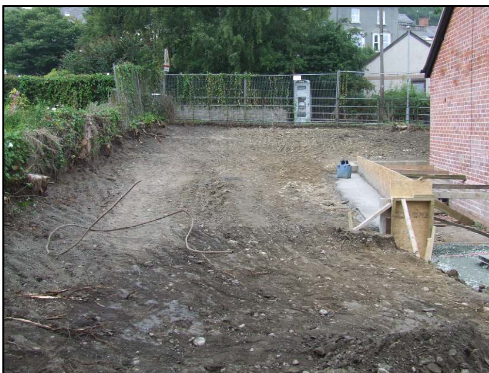
Photograph 2 Location from which surface soils elevated in PAHs have been removed, looking north west towards New Road
