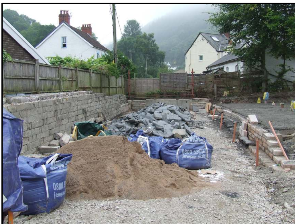
Photograph 8 Proposed location of track bed formerly occupied by soil mound (removed to canal wharf), looking south west
