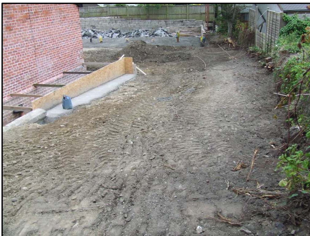
Photograph 3 Location from which surface soils elevated in PAHs have been removed, looking south east
