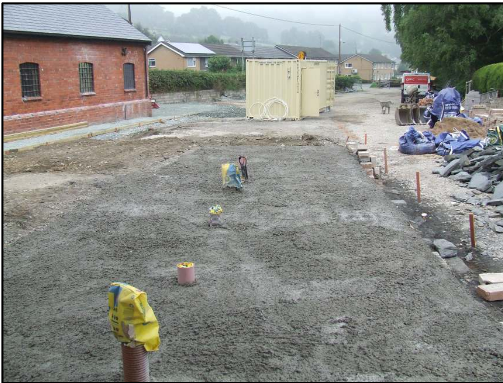
Photograph 9 Concrete capping to soil repository forming the station platform, looking north east
