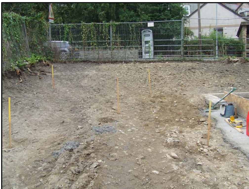
Photograph 5 Validation sampling points, looking north west
