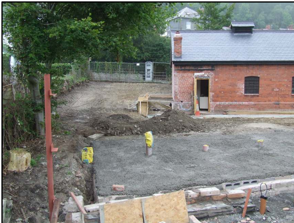
Photograph 1 Western end of the site showing station platform (soil repository) in foreground and area from which soils were removed beyond
