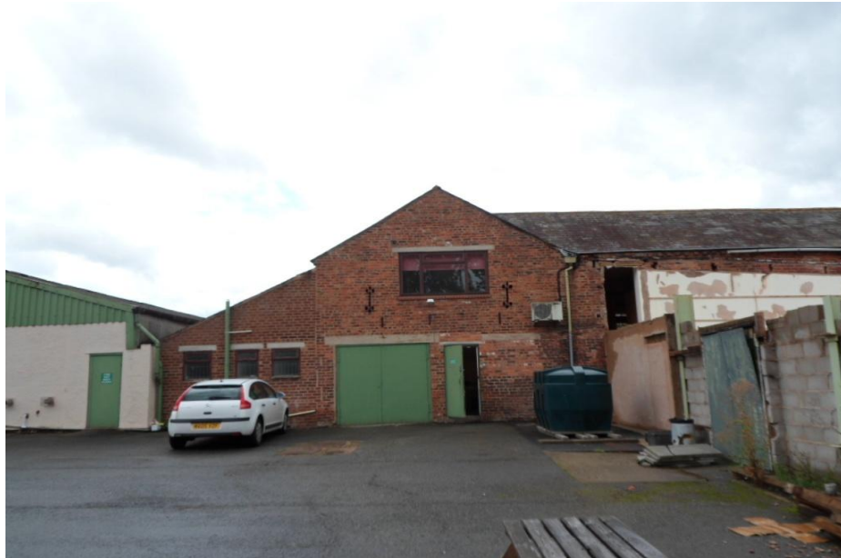
Existing eastern gable
