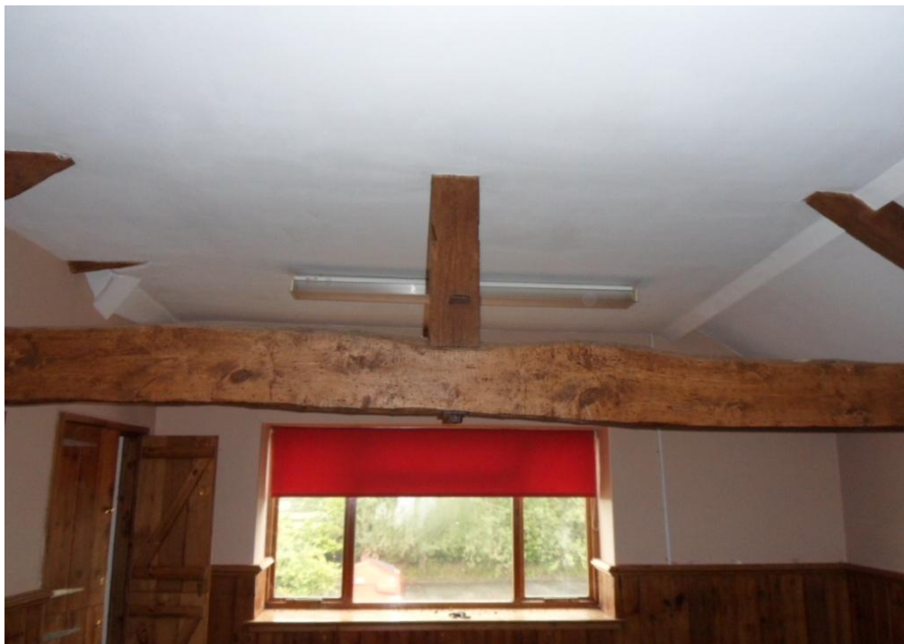
Example of existing King post truss, part obscured by inserted ceiling
