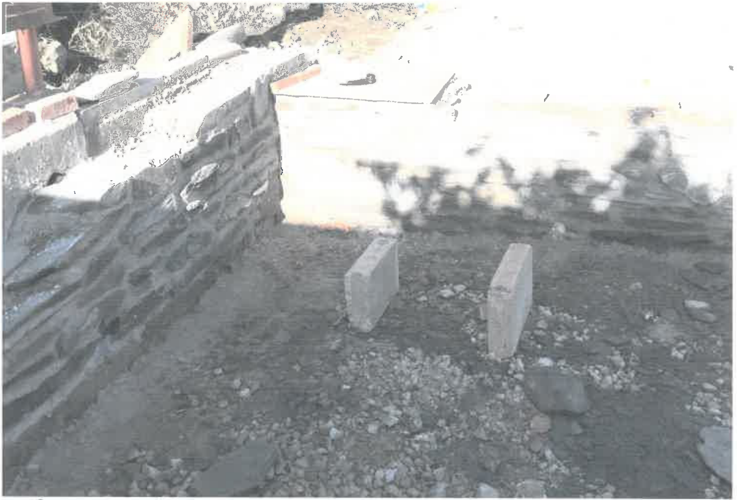
BUILDING PLATFORM IN FRONT OF BUND
