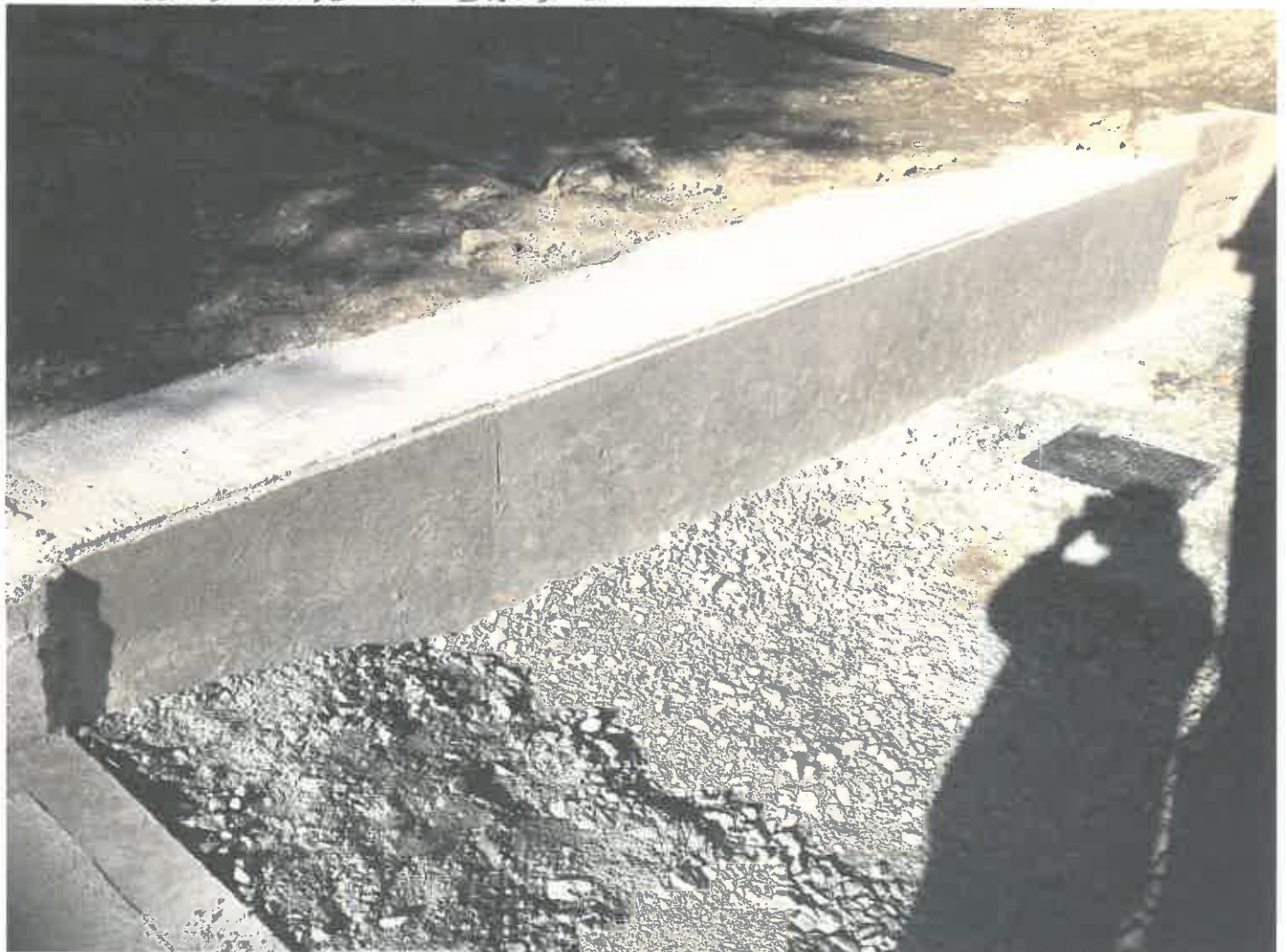
RETAINING WALL FINISHED ON BACK OF SHED
