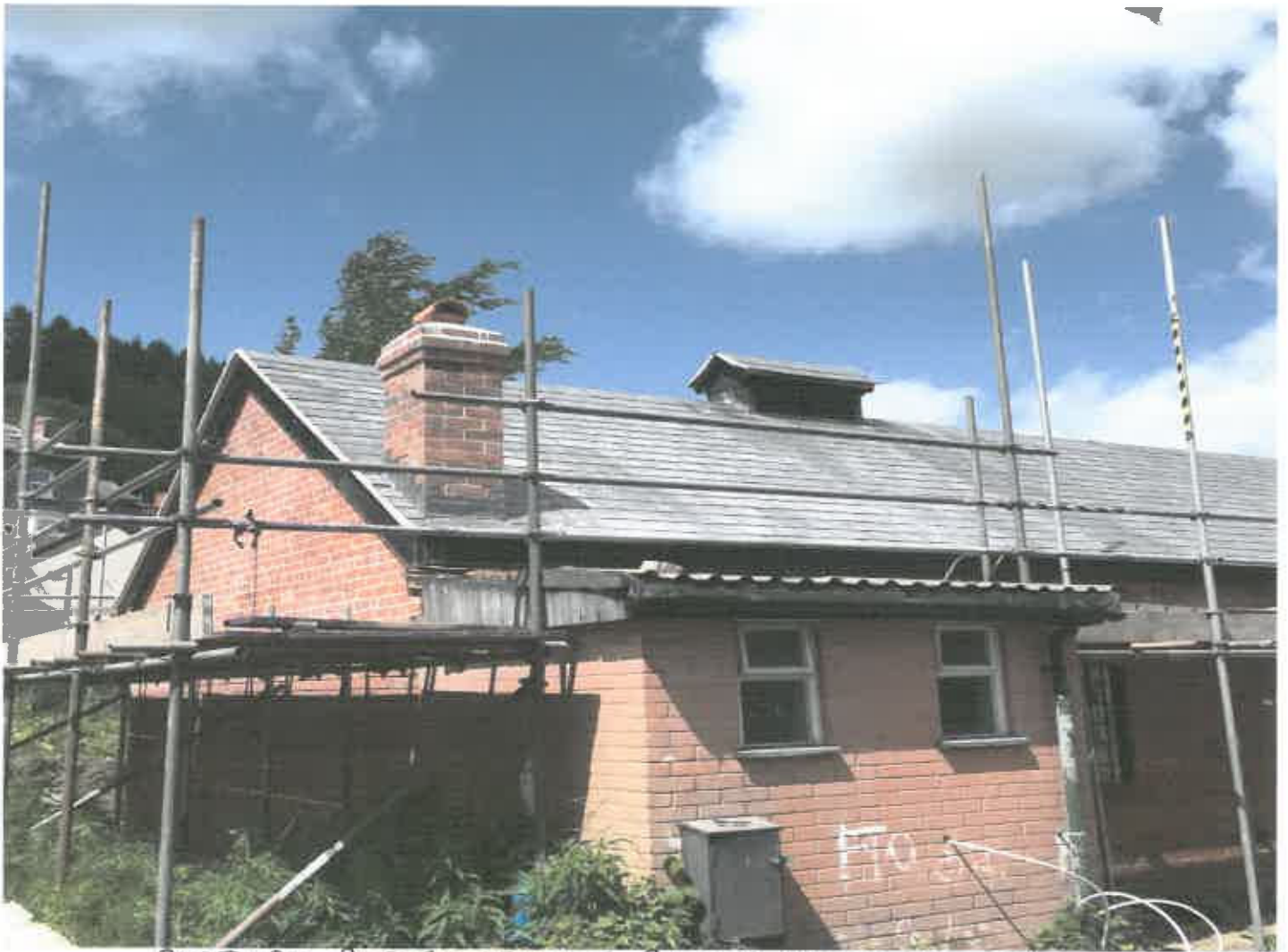
PICTURE BEFORE TOILET BLOCK CAME DOWN
