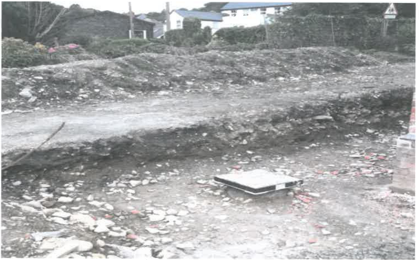
SEWAGE CONNECTIONS / SPOIL IN PILE WAITING FOR BUND
