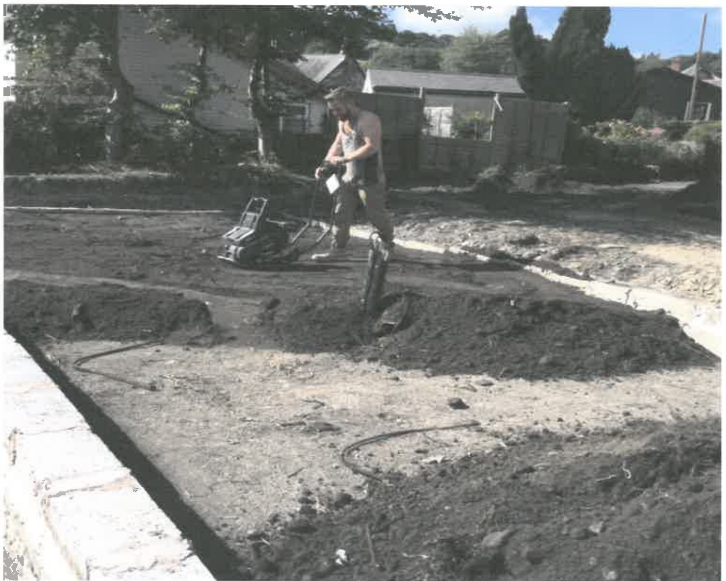
COMPRESSING SPOIL WITH WALKER PLATE
