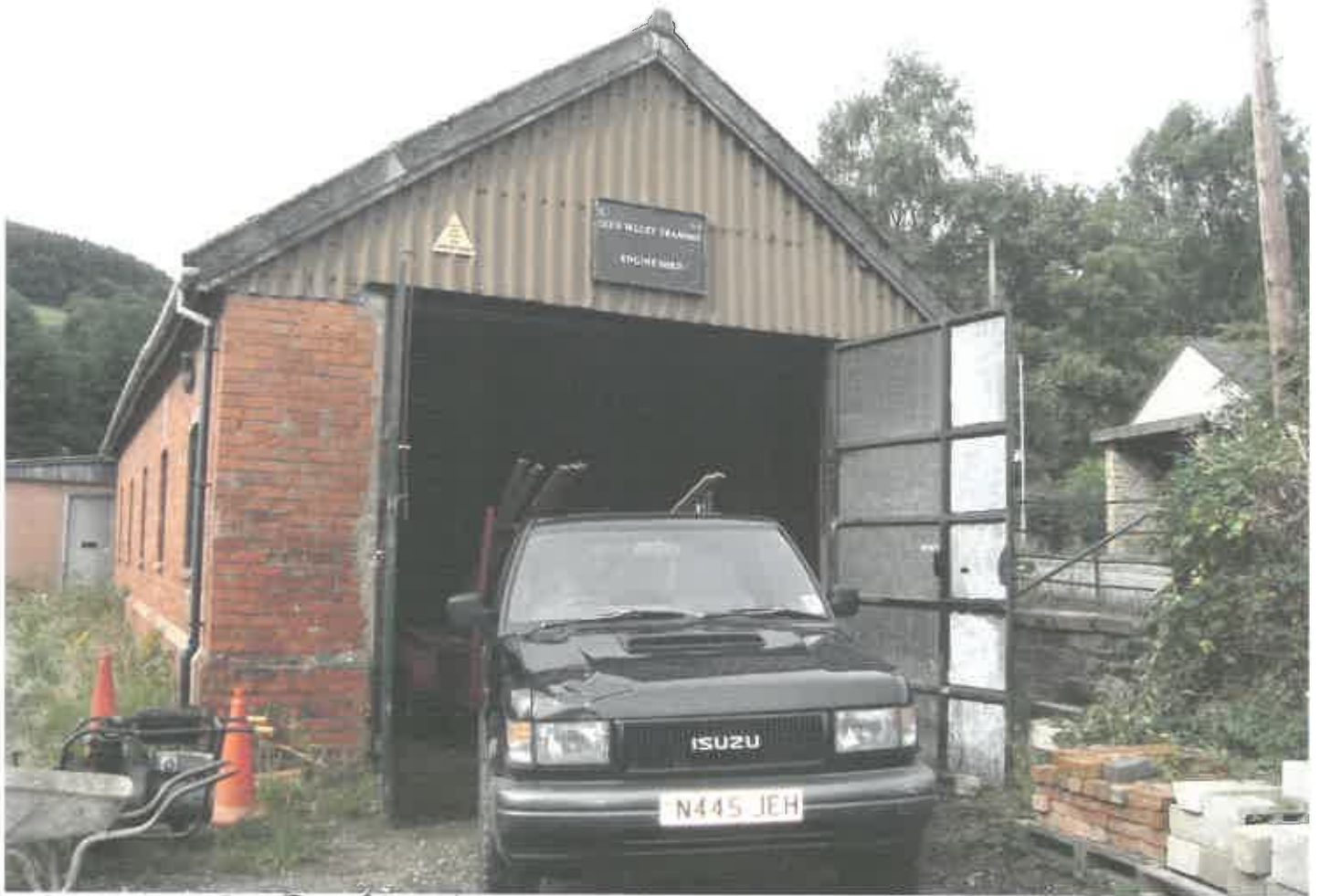
OUTSIDE SHED EARLY IN 2015 BEFORE WORK STARTED
