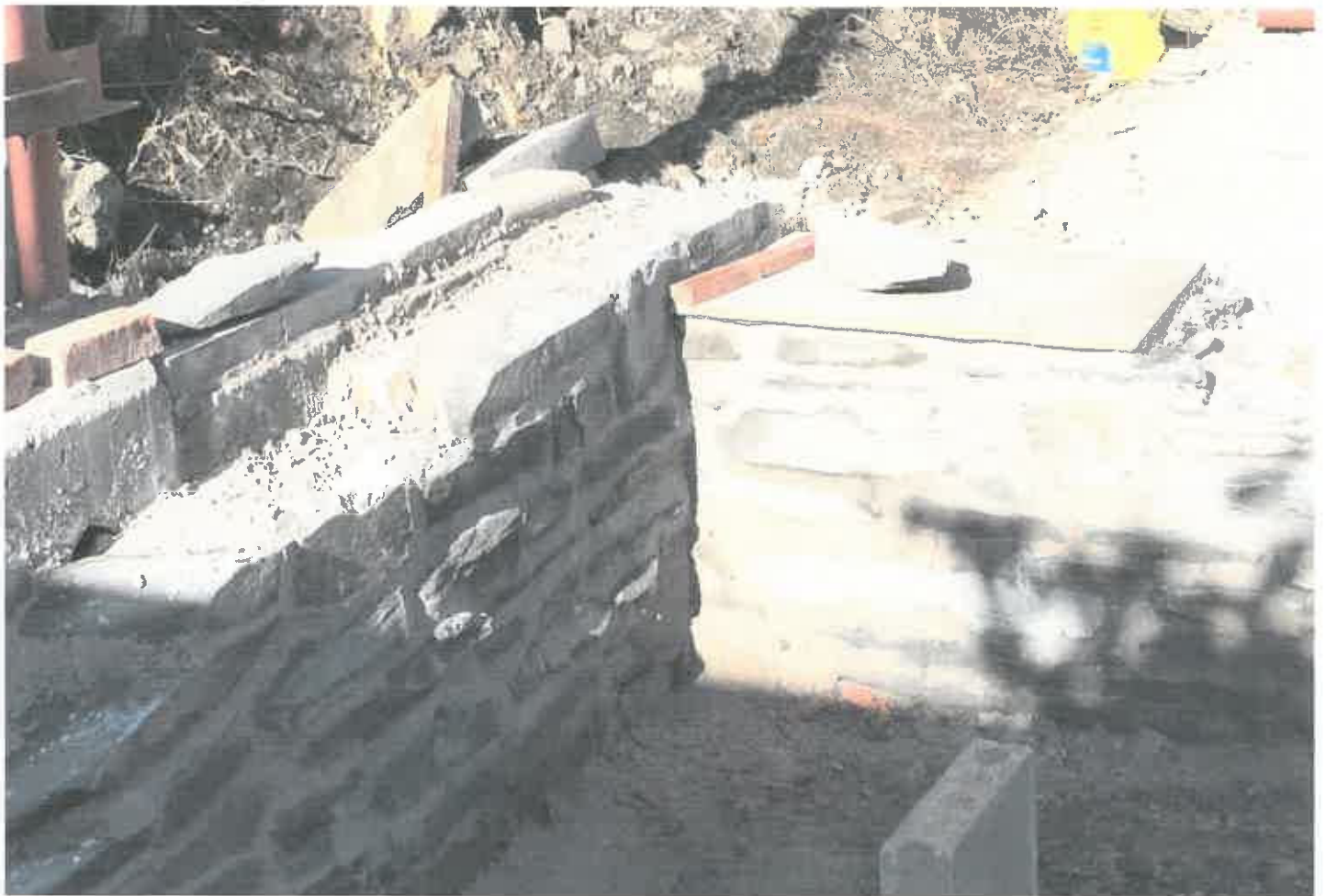
WELSH SLATE FRONT AS ORIGINAL.
