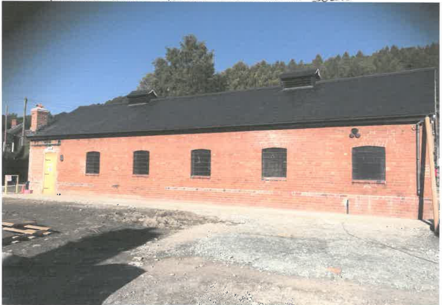
NEW ROOF / SMOKE VENTS / CHIMNEY / TOILET BLOCK REMOVED
