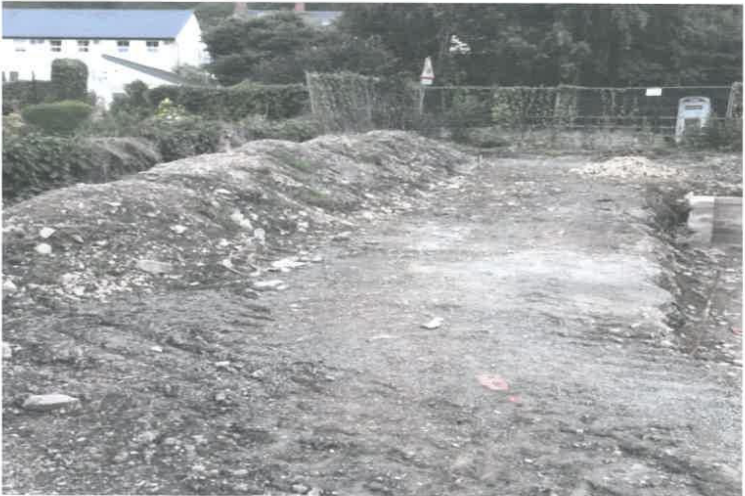
END VIEW OF SITE SHOWING RETAINING WALL.
