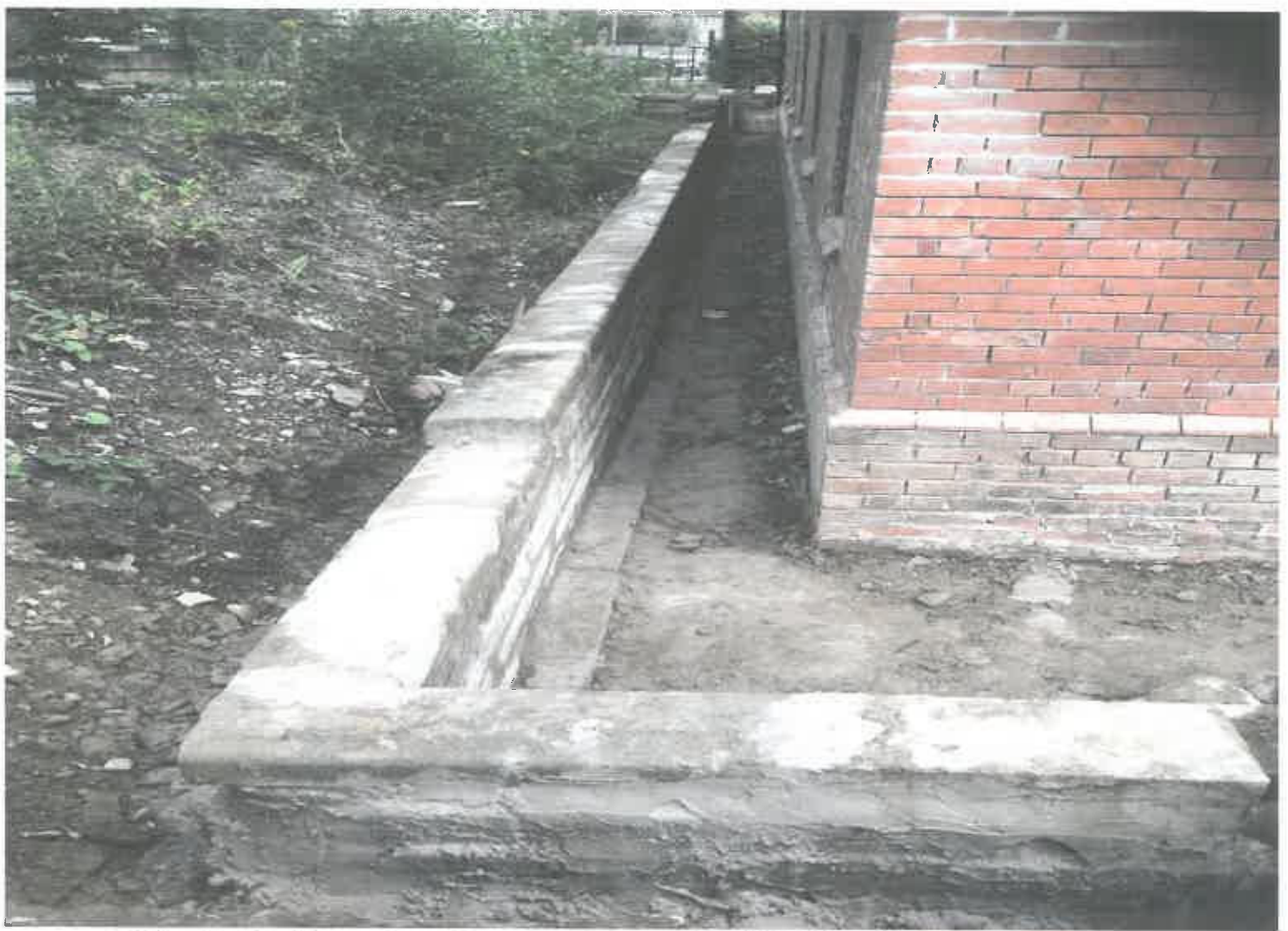
ROAD SIDE OF SHED SHOWING RECYCLED BLOCKS
