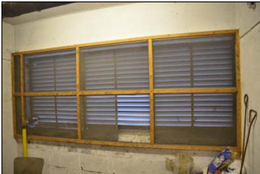
8. Missing grill section in the boiler room
