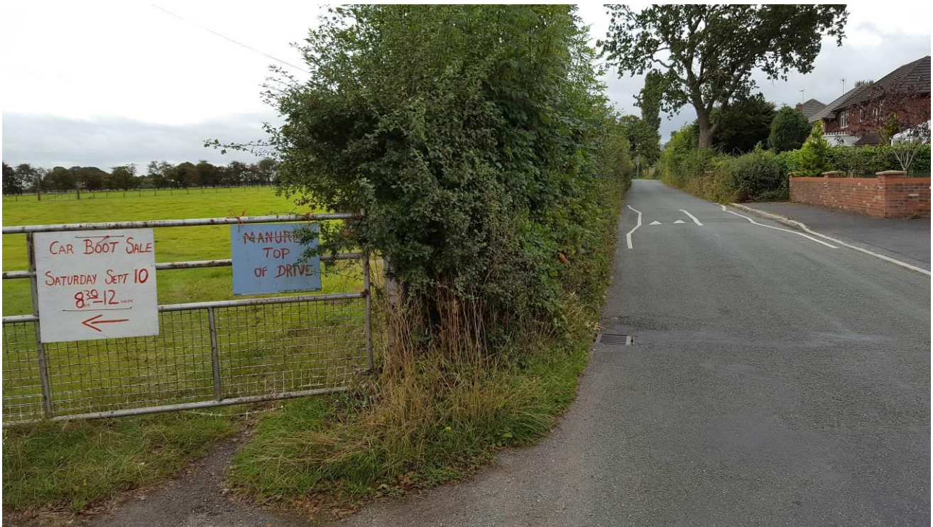
Photo 3 – Existing site access gate looking south along Gamford Lane. Note road gully on left hand side of road
