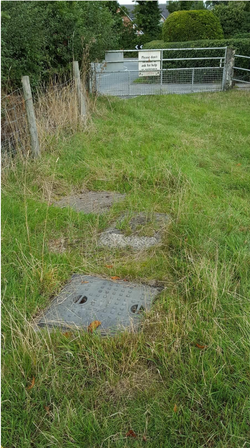
Photo 2 – Service manhole covers at the main northern access gate, adjacent to junction of Gamford and Darland Lane
