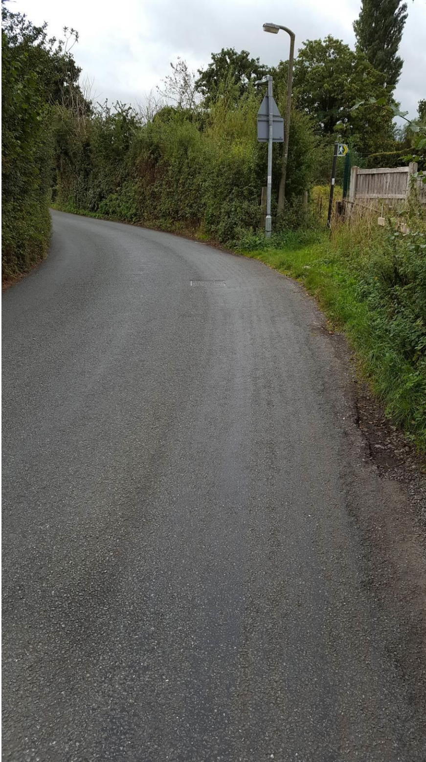
Photo 4 – Service manhole covers at the main northern access gate on Gamfrod Lane
