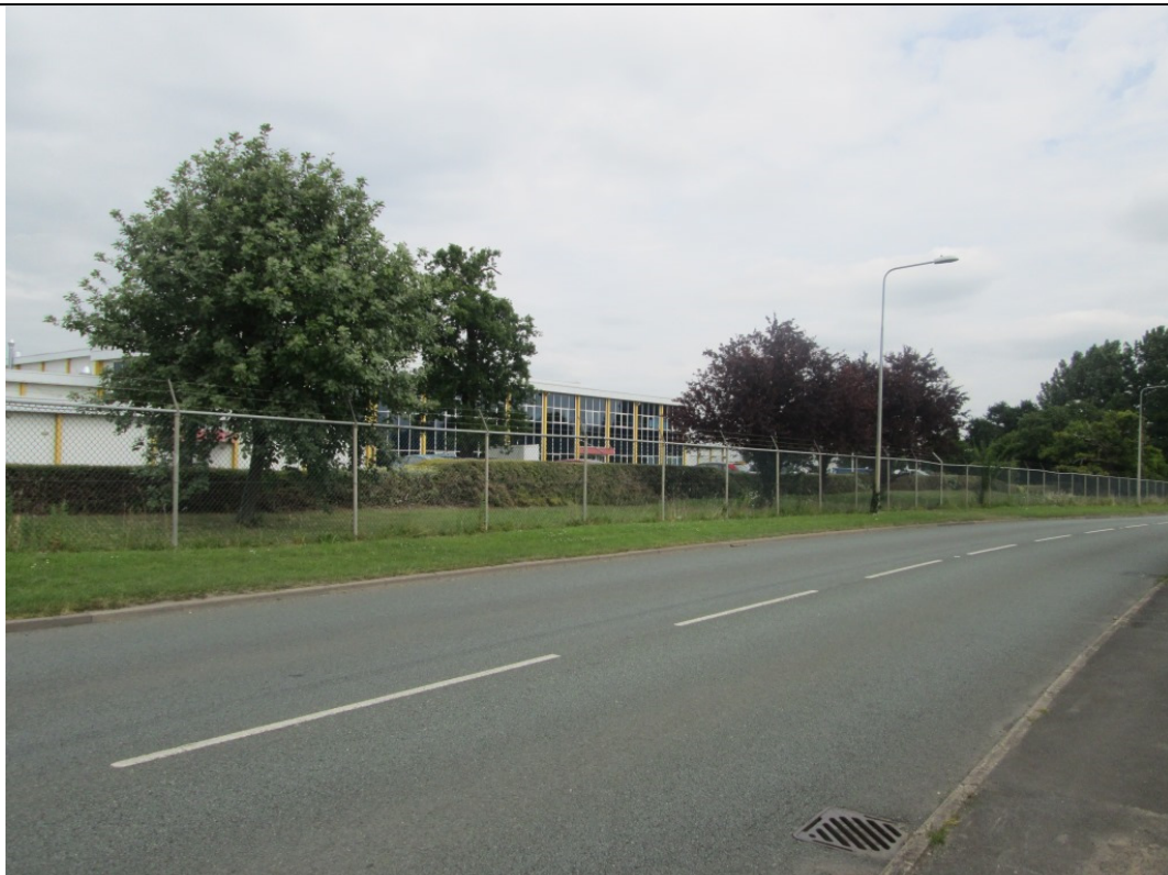
Photograph: 10 | Adjacent unit to the east of the Subject Property (view north east)
