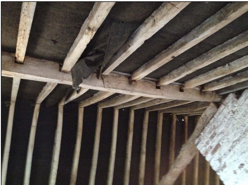
A1.12 Plate 12 – Building B3 Roof structure and potential roosting features
