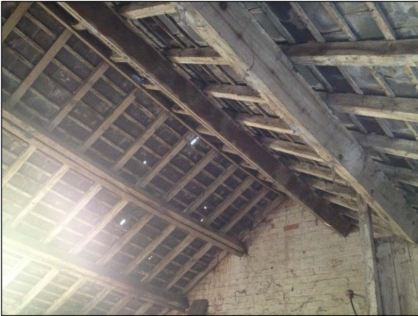
A1.9 Plate 9 – Building B2, roof structure
