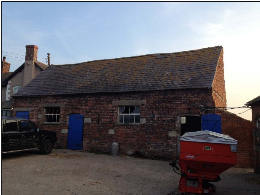
A1.5 Plate 5 – Northern elevation of Building B3
