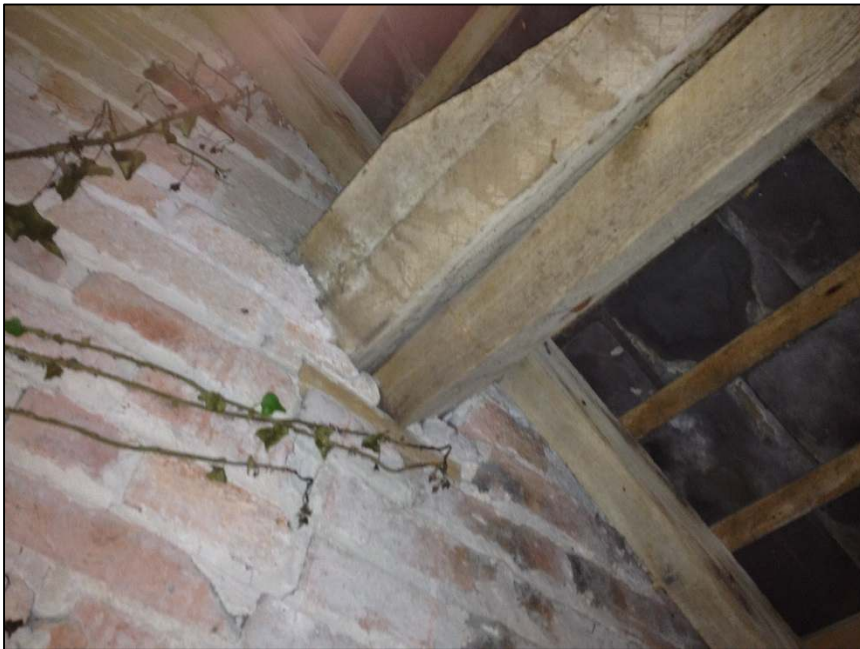
A1.8 Plate 8 – Example of potential roost location within Building B1a
