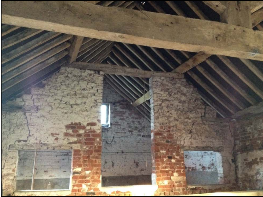
A1.11 Plate 11 – Building B3 roof structure
