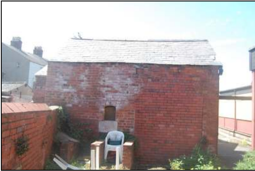
16. Sealed areas under the front gable of the coach house
