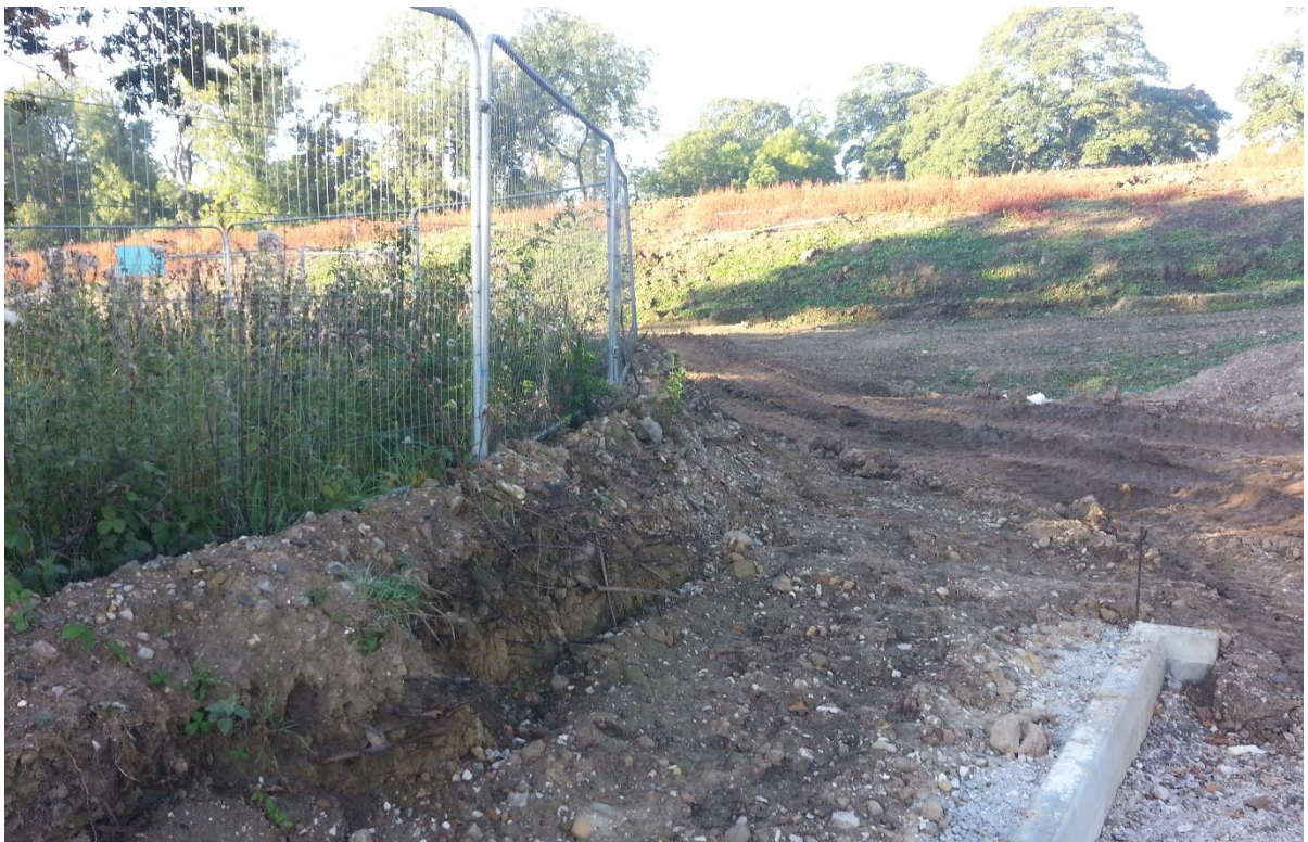
Small roots visible in bottom left are remains of Group G4 removed as part of the planning application.
