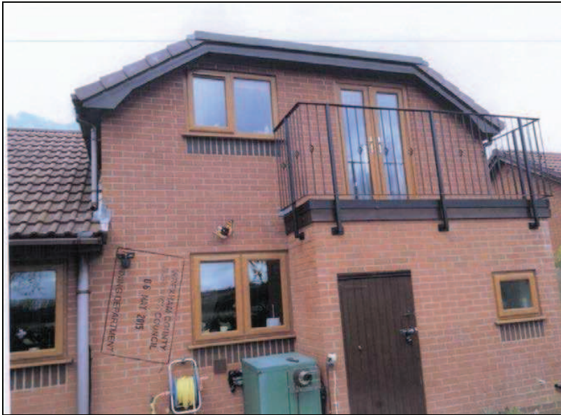
Balcony as built
