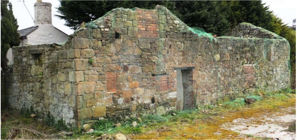
Building Exterior. Left: Northeast elevation. Centre and right: Northwest elevation.
