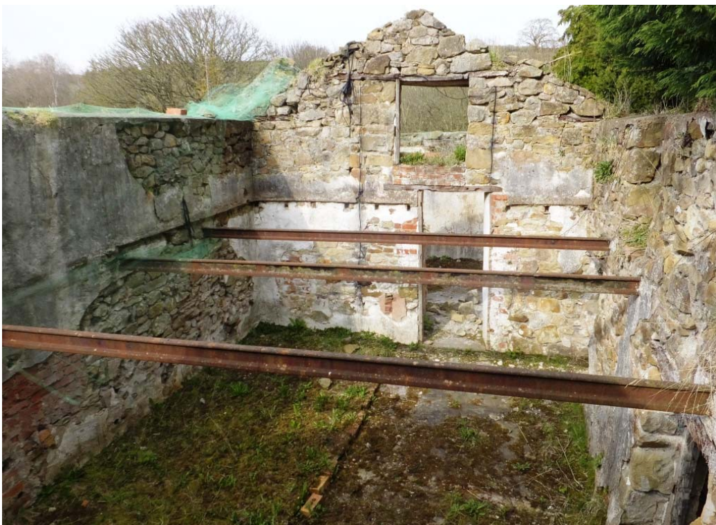
Building 'Interior'. View of the southwest-end room. Looking northeast from southwest.
