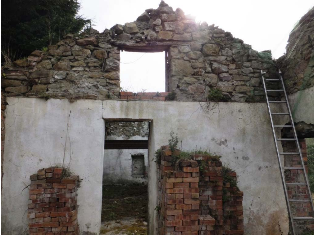
Building 'Interior'. View of the northeast-end room. Looking southwest from northeast.
