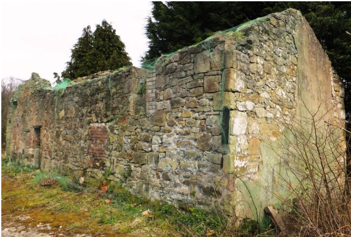
Building Exterior. Left and centre: Northwest elevation. Right: Southwest elevation.
