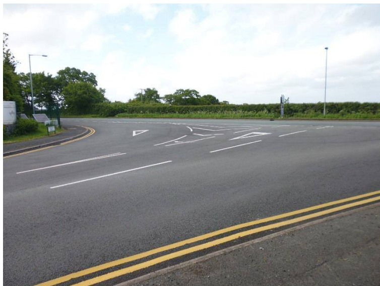
Photo 2: Davy Way / Rackery Lane Priority Junction
