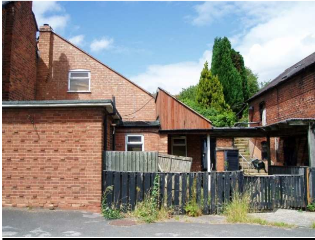
Photograph 5. Gredington Arms – pub roof void
