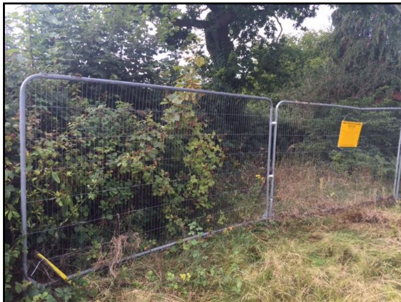
Photos 1 – Weldmesh tree protective fencing erected in correct location around tree number 2
