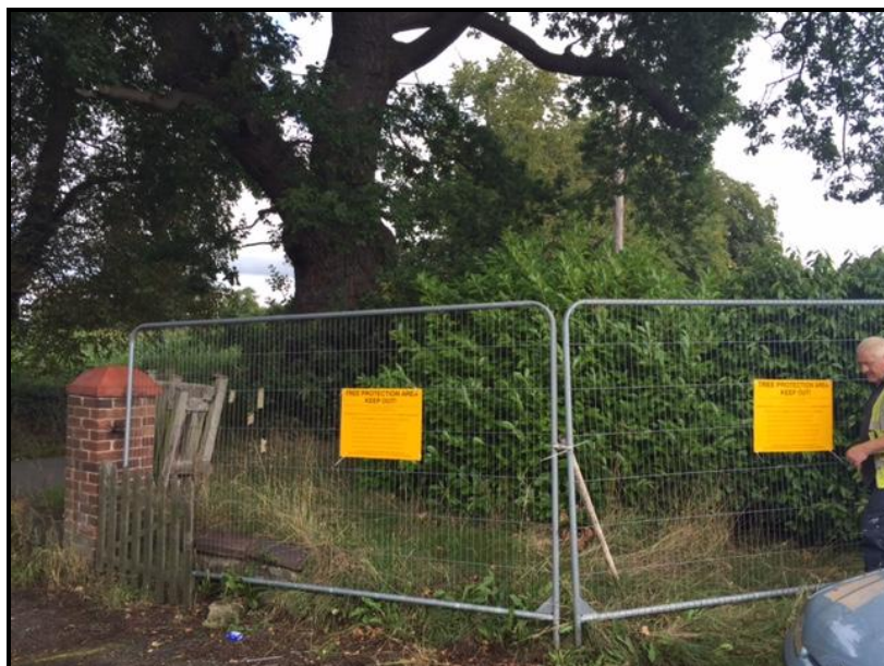
Photo 3 - Protective fencing around tree number 1. Existing access driveway to be left in situ for ground protection
