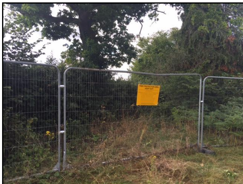
Photo 2 - Tree protective fencing with signs affixed to fence panels around tree number 2
