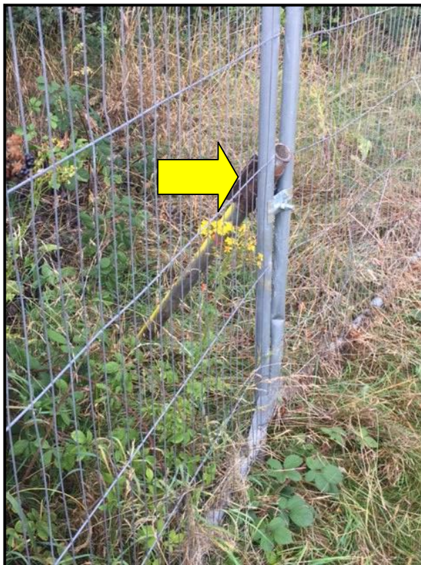
Photo 4 - Scaffold pole driven into ground to prevent movement of panels
