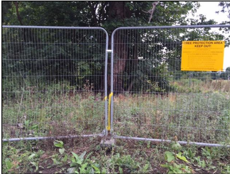
Photo 7 - Scaffold pole driven into ground of fencing to Pine tree to east
