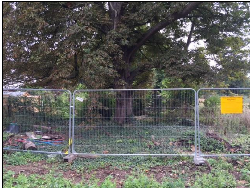
Photos 1 – Weldmesh tree protective fencing erected in correct location around Horse Chestnut tree at site entrance
