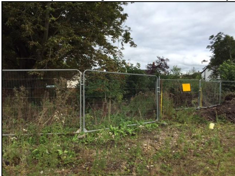
Photo 5 - Tree protective fencing with signs affixed along SW boundary
