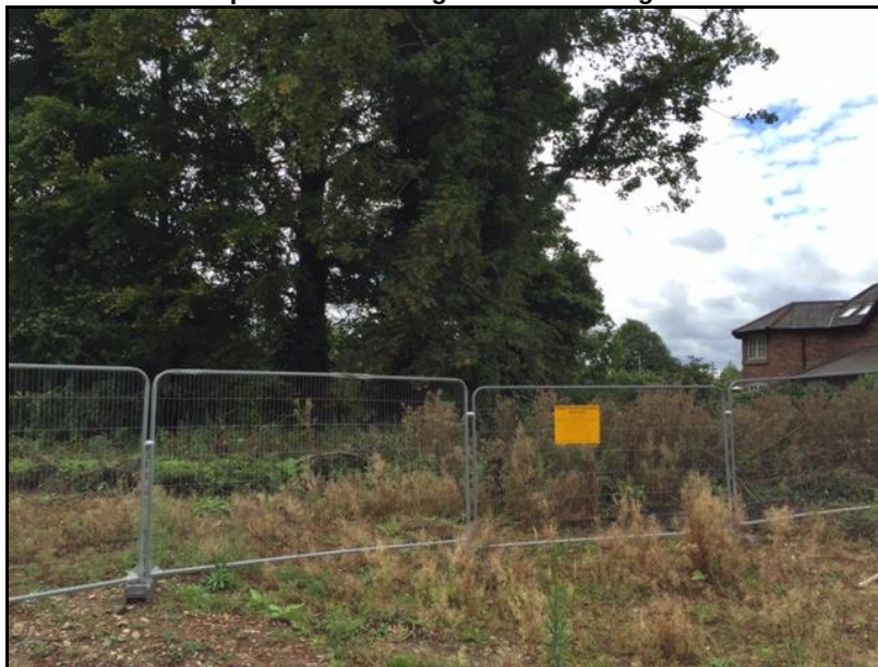
Photo 8 - Tree protective fencing with signs affixed erected around trees to south
