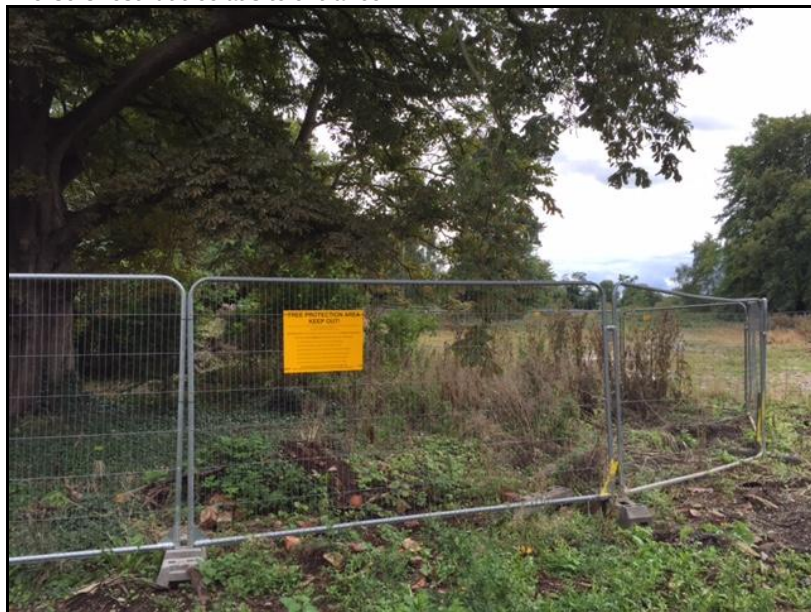
Photo 2 - Tree protective fencing with signs affixed to fence panels
