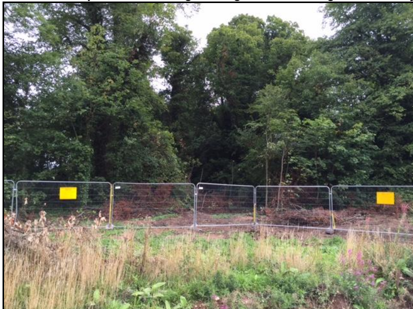
Photo 6 - Tree protective fencing with signs affixed around trees to NE
