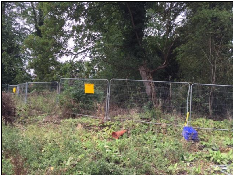
Photo 4 - Tree protective fencing around wooded area to western boundary
