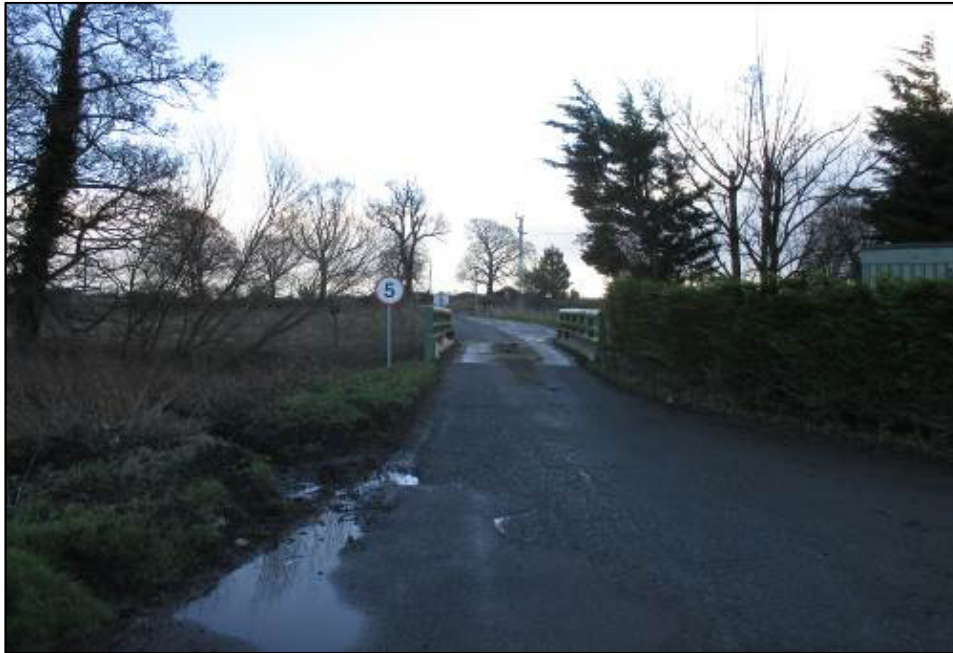
Photo 2.3: View of Bridge from Cefn Road
