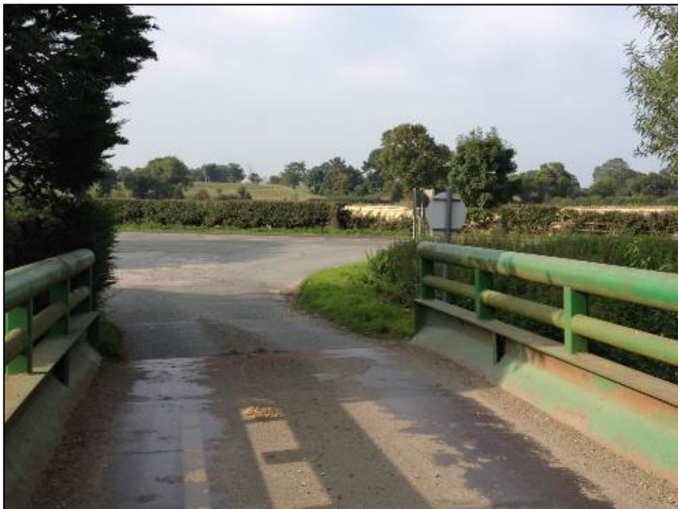
Photo 2.4: View from Bridge (looking back to Cefn Road)
