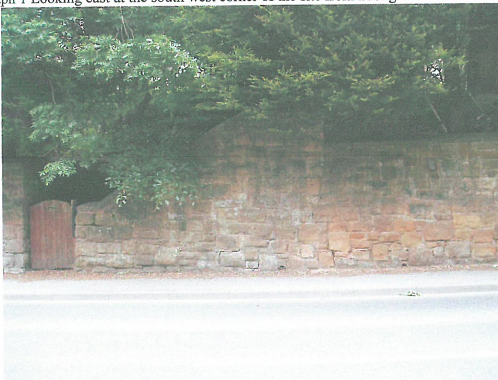
Photograph 2 looking east at the retaining wall on the western boundary, from Broughton road
