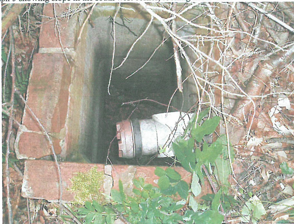
Photograph 6 showing drain in the south west corner of the site.
