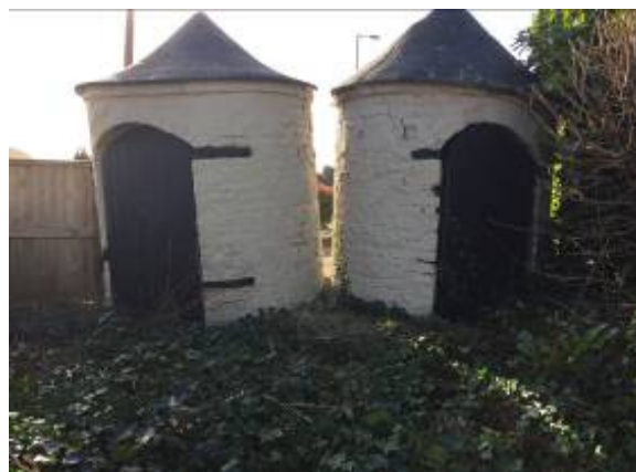
Adjacent “Privies” located to the west of the building
